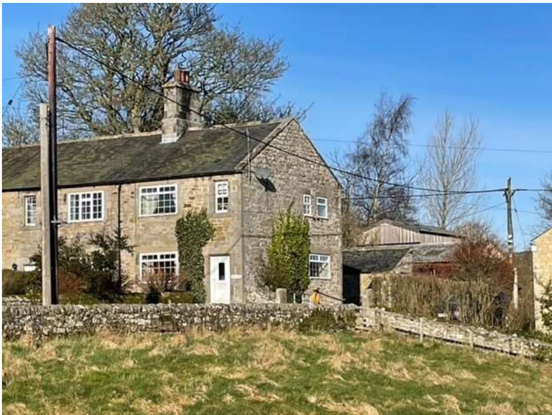
Ivy Cottage – SE view
