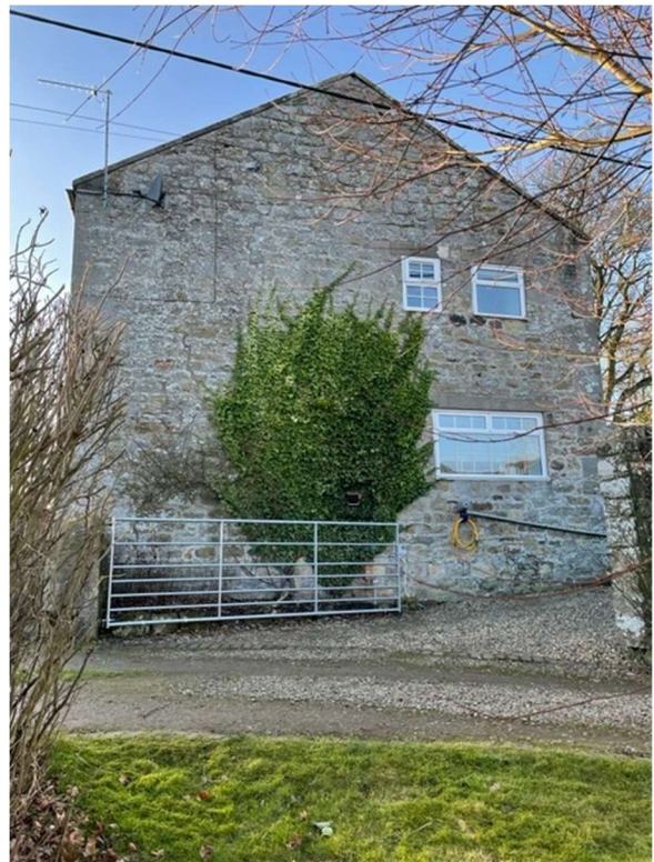
Ivy Cottage - east elevation
