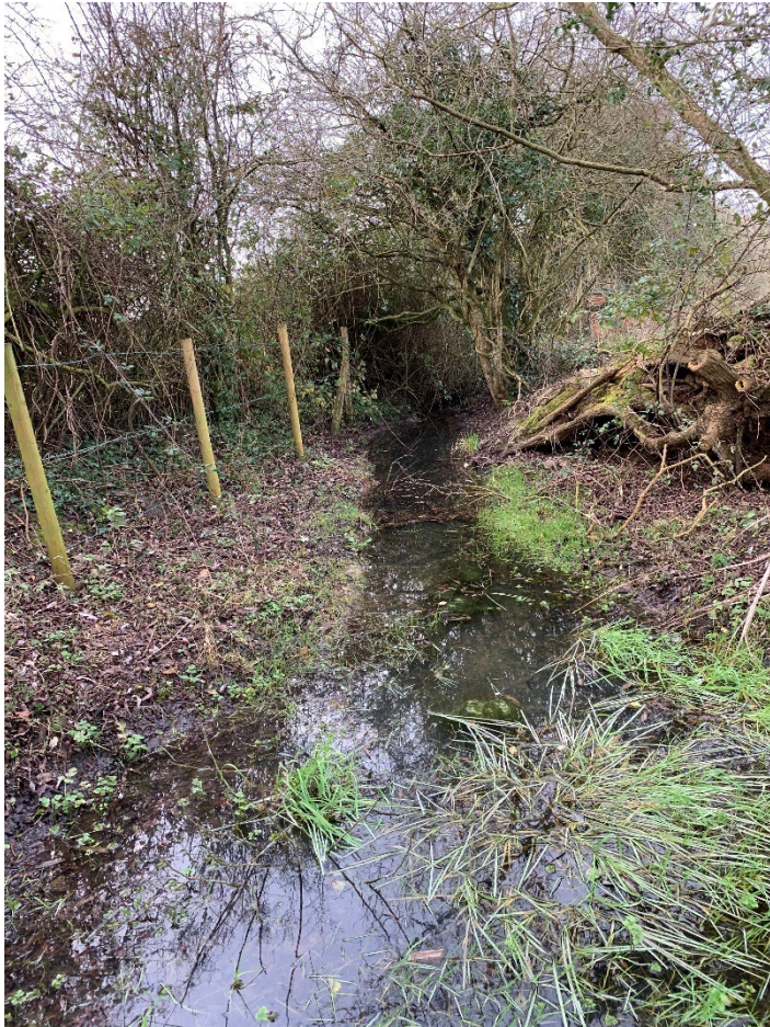
Photograph 9. Section of offsite drainage ditch.
