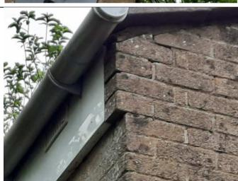
Area of missing mortar under the corner tile and adjacent to the fascia at the south western corner of the building. Approximately 2cm x 4cm in size.
