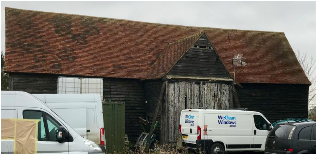
Fig.13: Southwest elevation, Brick House Farm Barn.
