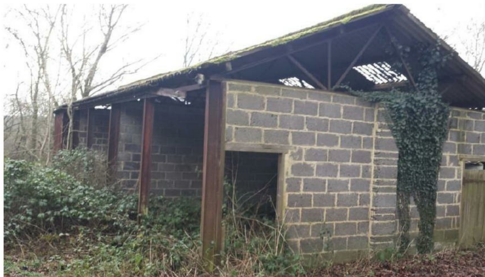
Image 1: Photograph of original building taken on 18 th January 2014
