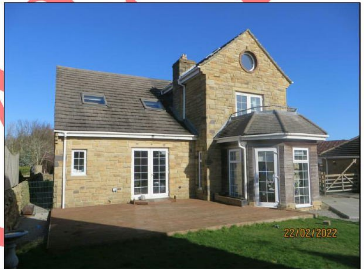
Figure 12. Main house, rear (southern) elevation, showing conservatory proposed for demolition.
