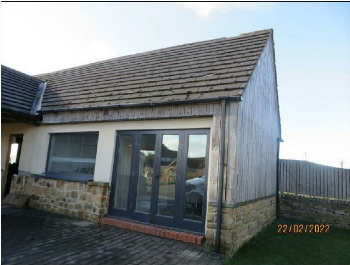
Figure 23. Outbuilding - 'Granny annex', showing wooden cladding.
