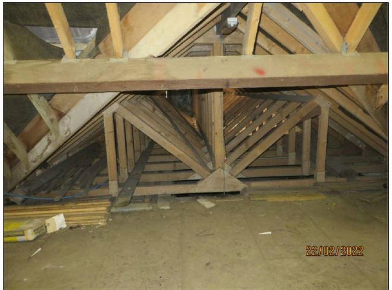
Figure 32. Roof void above stable bays.
