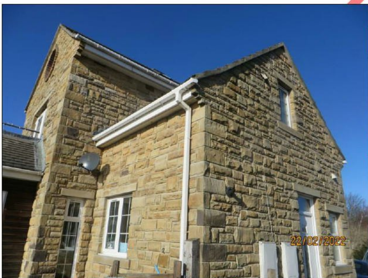
Figure 15. Rear (southern) and side (eastern) elevations.
