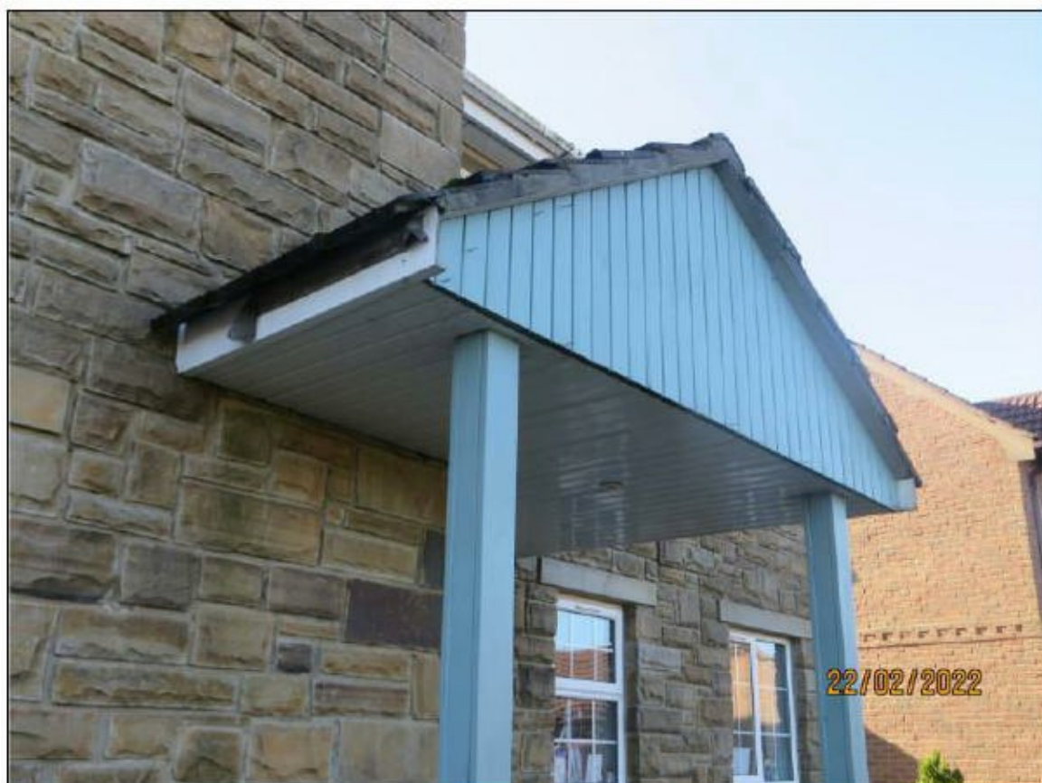
Figure 16. Covered portico on front elevation.
