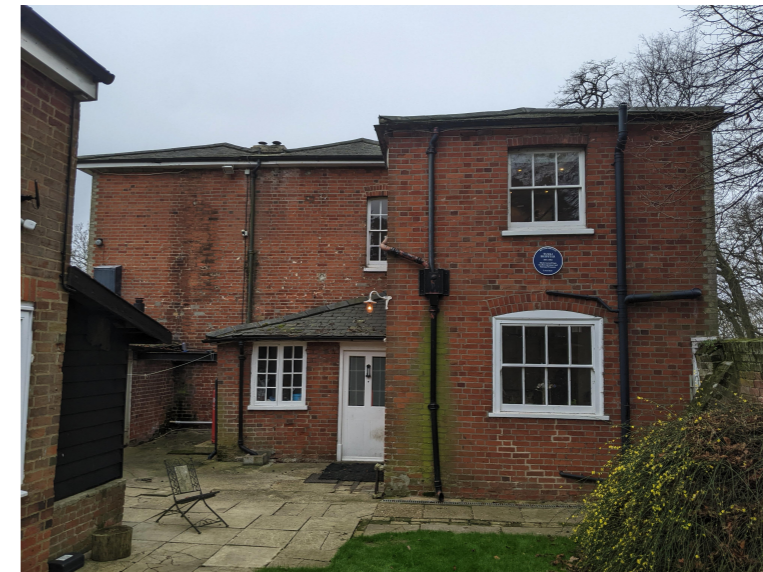
4. Existing north elevation, viewed from courtyard
