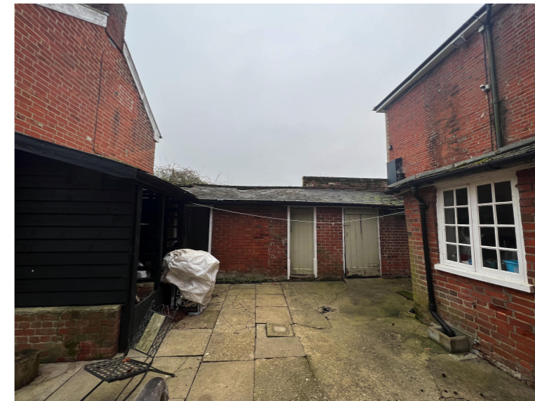
5. Existing courtyard, site of proposed extension
