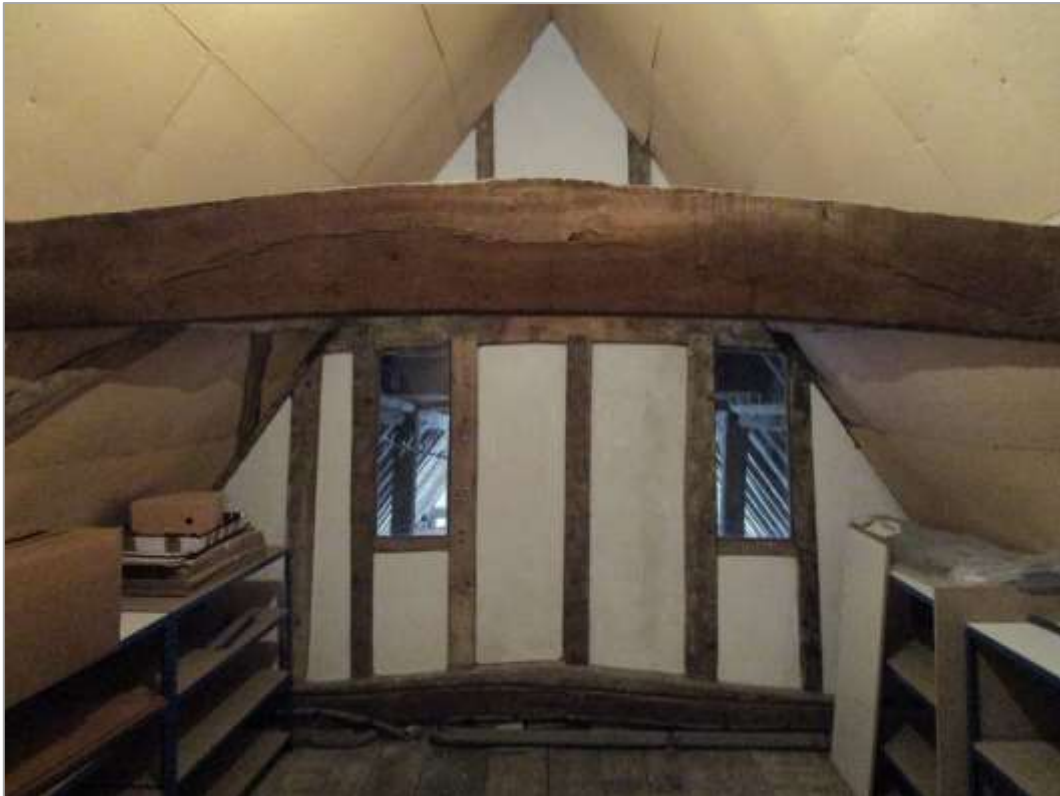
Fig. 44: A second view of the second floor space at the back of the main range, where it is proposed to form a bathroom. The roof timbers will be exposed, with insulation provided between. The boarded floor will be retained with a raised floor for the bathroom, to conceal the plumbing and spread the additional load of the bath.
