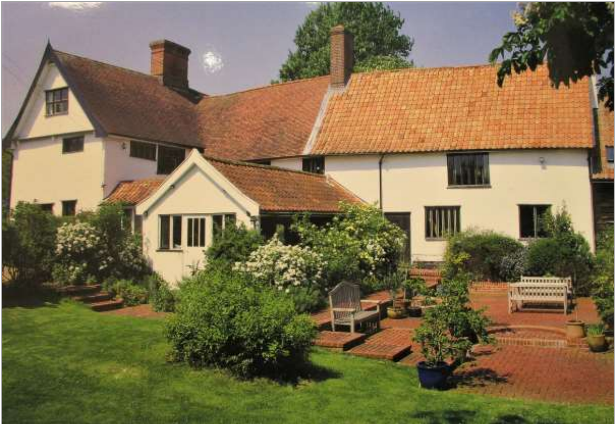
Fig. 27: Photograph from Jackson-Stops & Staff sales brochure, 2009, showing the new (1993) link between the utility room and kitchen and new brick terrace to south of former barn. The lower right hand window in the barn is probably that installed in 1979 (see para. 2.12) (SPAB file)
