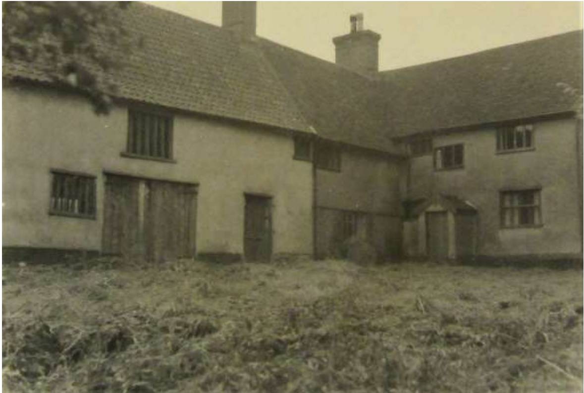
Fig. 10: The rear elevation of the front range and the north elevation of the barn, at the time of the SPAB's acquisition in 1965. By this time the weatherboard on the barn had been replaced with cementitious render. Note the door at the top end of the barn (SPAB file)
