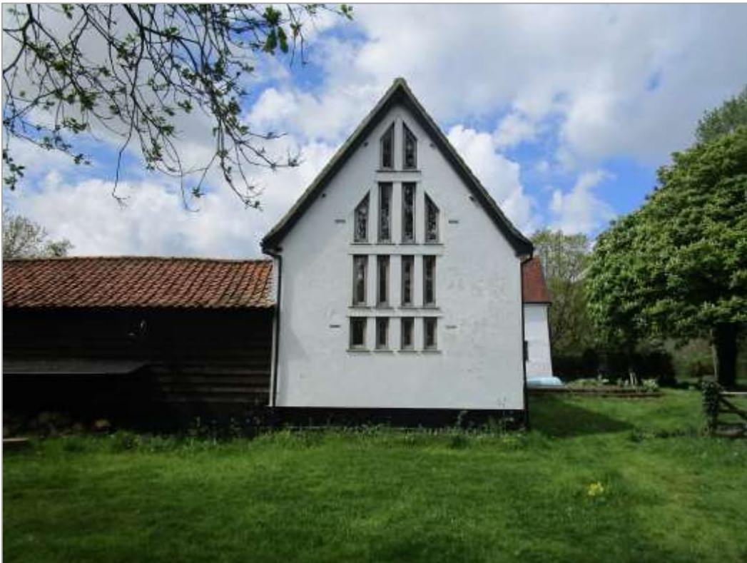
Fig. 31: East elevation of the lower former farm building, converted to residential use in 1998, when the present 'ecclesiastical' glazing was installed between the timber studs. These openings will be simplified and the detailing refined under current proposals.
