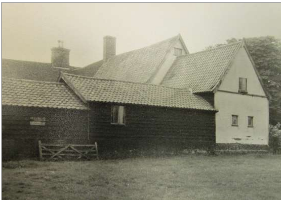
Fig 12: Photo with verso inscription 'Back of barns and outbuildings, July, 1965'. The weatherboard survived in part on the southern return of the eastern outbuilding and beneath plaster on the eastern gable end elevation. Note windows on this elevation and high level window in barn gable (SPAB file).
