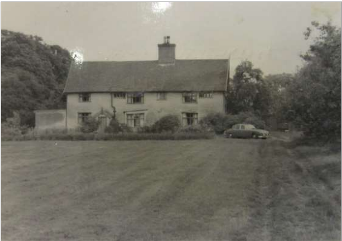
Fig. 9: Wingfield Priory in 1965, at the time of the SPAB's acquisition. The old lime render had been replaced with a more cementitious render. The lean-to structure to the east may have been that shown on the nineteenth century plans and maps (SPAB file)
