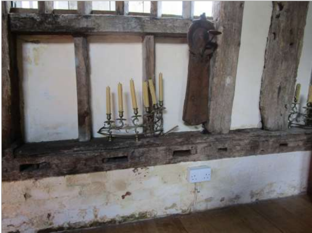
Fig. 40: Re-used sole plate and studs in the centre bay of the former barn, south side
