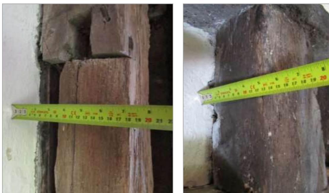
Figs 45 and 46: Typical variations in depth of studs in former barn
