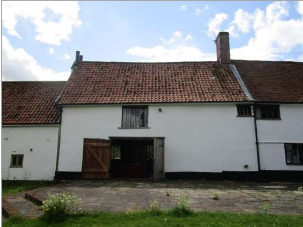
Fig. 30: North elevation of the former barn. Since 1990 (fig. 20) a door opening to the right has been blocked, and the barn doors replaced. Under current proposals the blocked opening will be partially re-opened as a mullion window and new barn doors provided.
