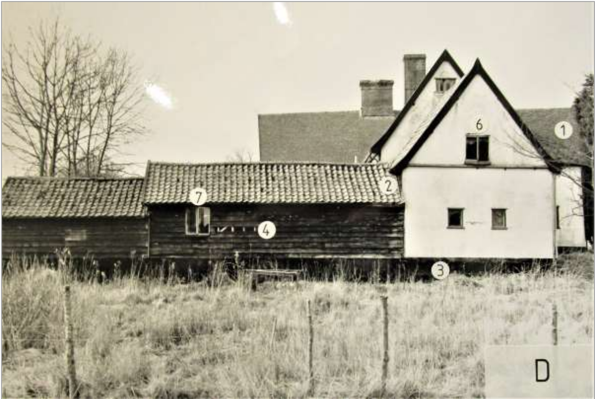
Fig. 21: View from east, 1990 (SPAB file)
