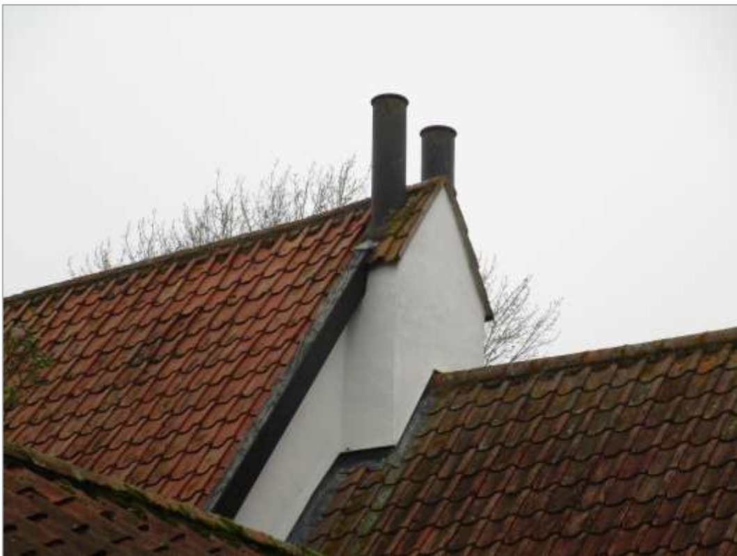
Fig. 33: The external stack on the east gable end of the former barn was built in 1998; it will be retained to house the heating flues.
