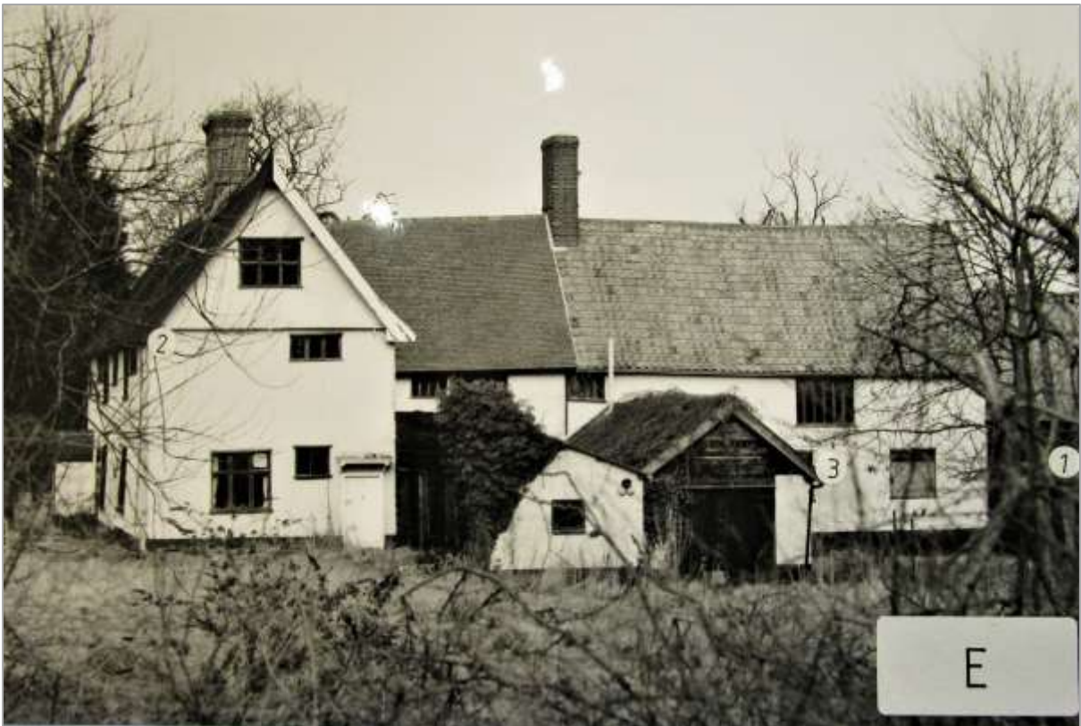
Fig. 22: View from south, 1990 (SPAB file)
