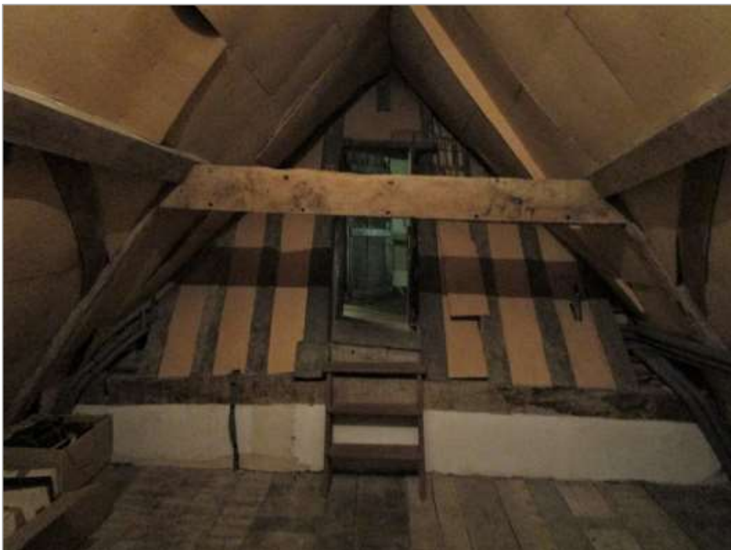
Fig. 43: Steps down from the second floor landing to the proposed bathroom.
