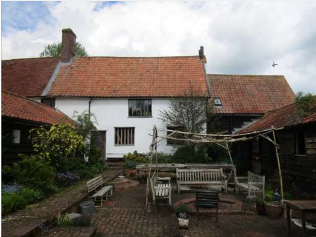
Fig. 32: South elevation of the former barn. The door shown to the left of the mullion window will be blocked and the brick plinth and sole plate reinstated. Central barn doors will be reinstated (as shown on old plans and as evidenced by the fabric). The plate glass casement window lower right dates from 1979; it will be replaced by a diamond mullion window.
