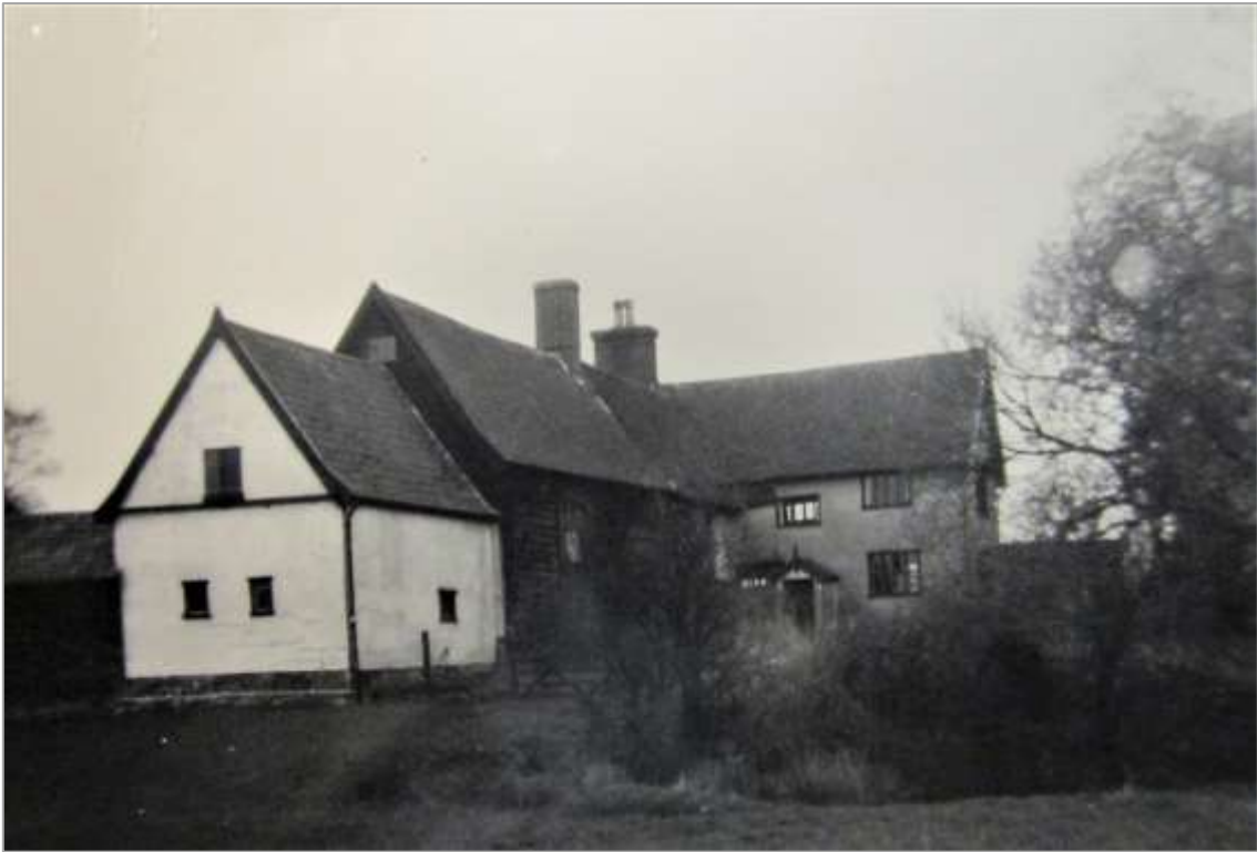
Fig. 8: Undated, probably mid-twentieth century photograph, showing the barn clad in weatherboard and the lower range to the east rendered, possibly over weatherboard (SPAB file)
