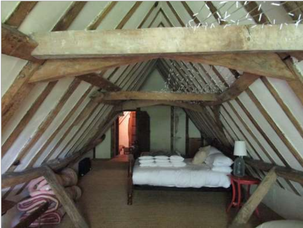
Fig. 42: The second floor guest bedroom. The far end will be partitioned off to create a small lobby and storage space.
