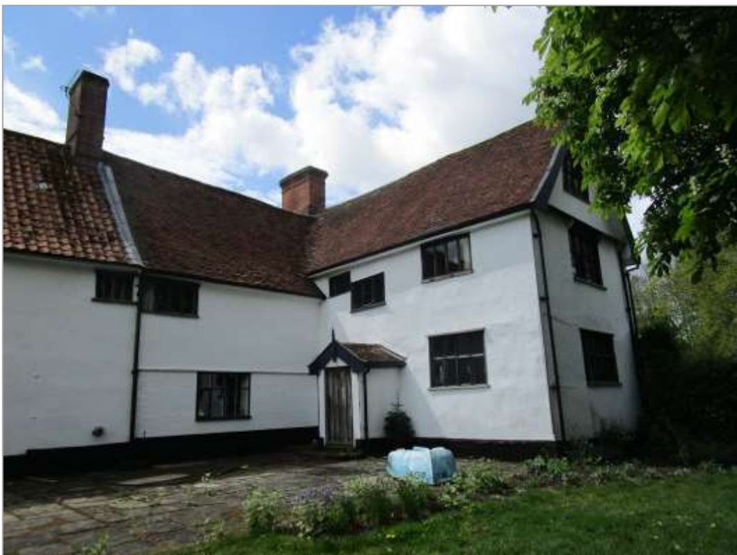
Fig. 29: The front range and former dairy form a T-plan; the attached former barn (with pantiles) is to the left.
