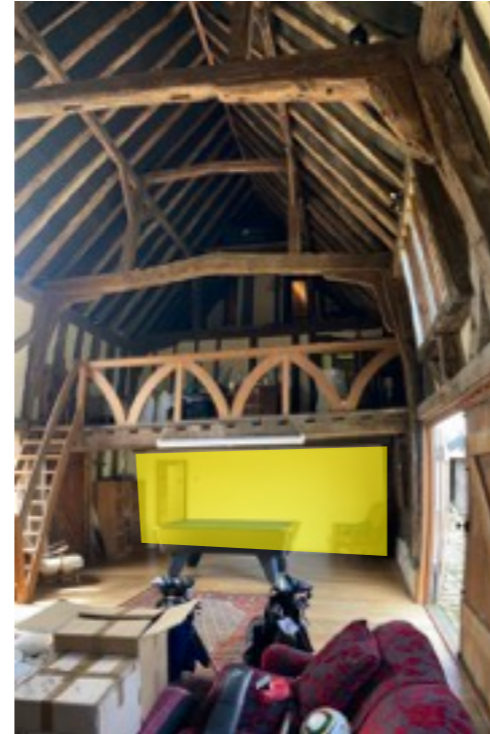
Yellow highlighted area shows wall to be removed.
