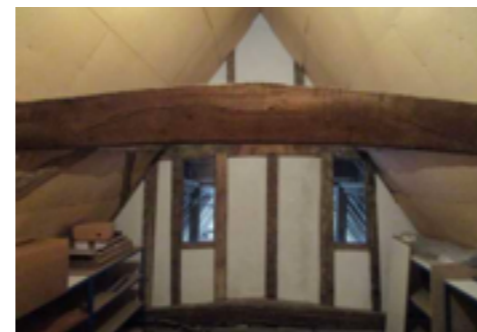
Second floor attic storage to be converted in a shower room.
