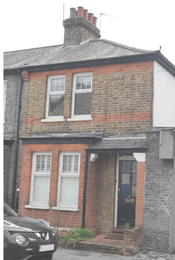
Existing Facade of Property
