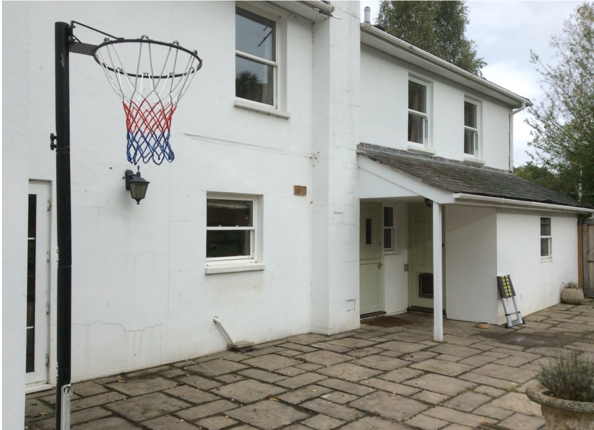
Figure 8. Eastern face of March House where the proposed extension is to be sited.
