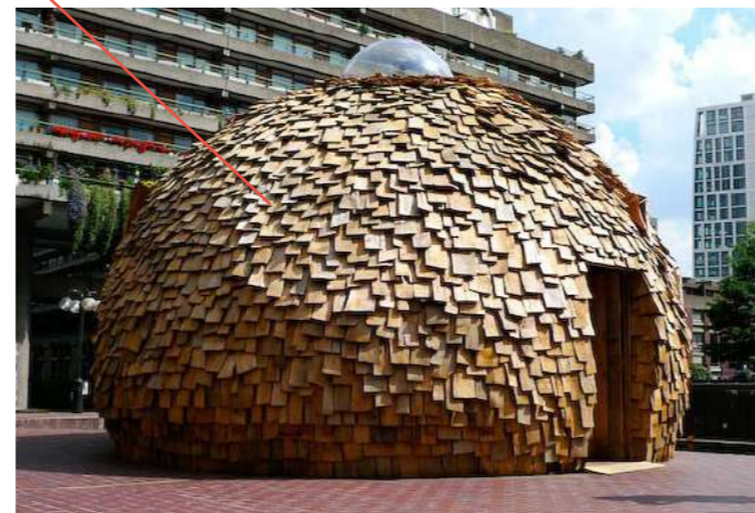
LEFT - ROUGH OAK SHINGLES FOR POD CLADDING, UNFINISHED LEFT TO SILVER.
