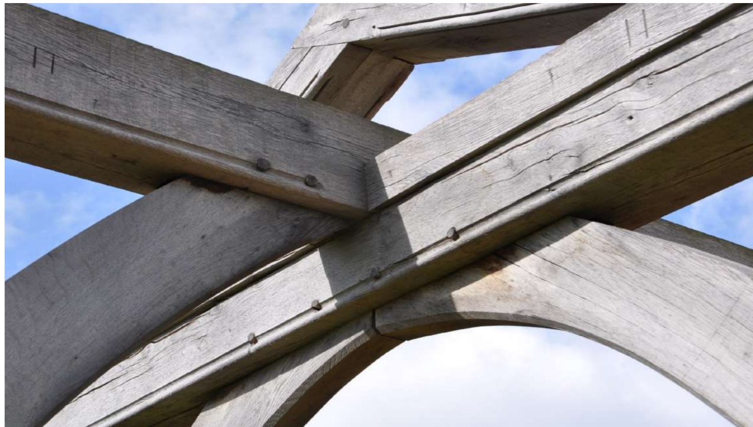
BELOW - OAK BEAMS WITH SIMPLE MOULDINGS TURNING SILVER GREY WITH TIME
