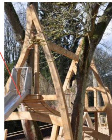
LEFT - STAINLESS STEEL SLIDE WOBBLE BRIDGE IN ROUGH SAWN GREEN OAK AND SYTHETIC HEMP COLOURED NETTING
