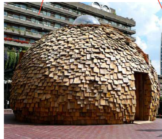
RIGHT - ROUGH OAK SHINGLED STRUCTURE
