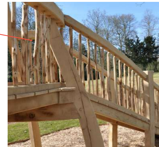
ABOVE - COPPICED CHESTNUT BALUSTERS WITH OAK DECKING AND FRAME.
