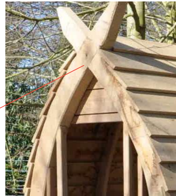
RIGHT - TRADITIONAL JOINERY IN ROUGH SAWN UNFINISHED GREEN OAK
