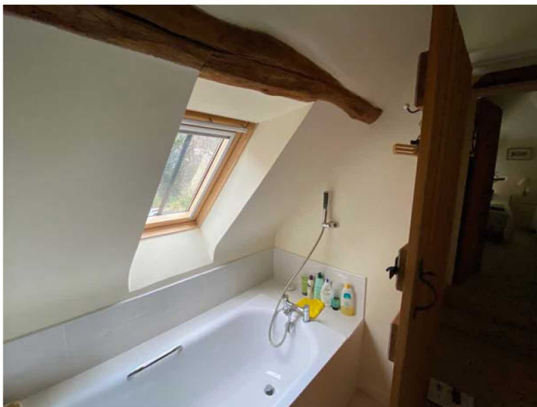
Above: Existing rooflight over bathroom
