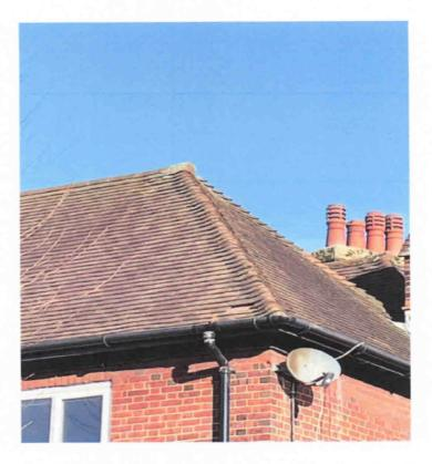
Existing roof tiles to be removed, set aside and re-used as covering for new mansard
