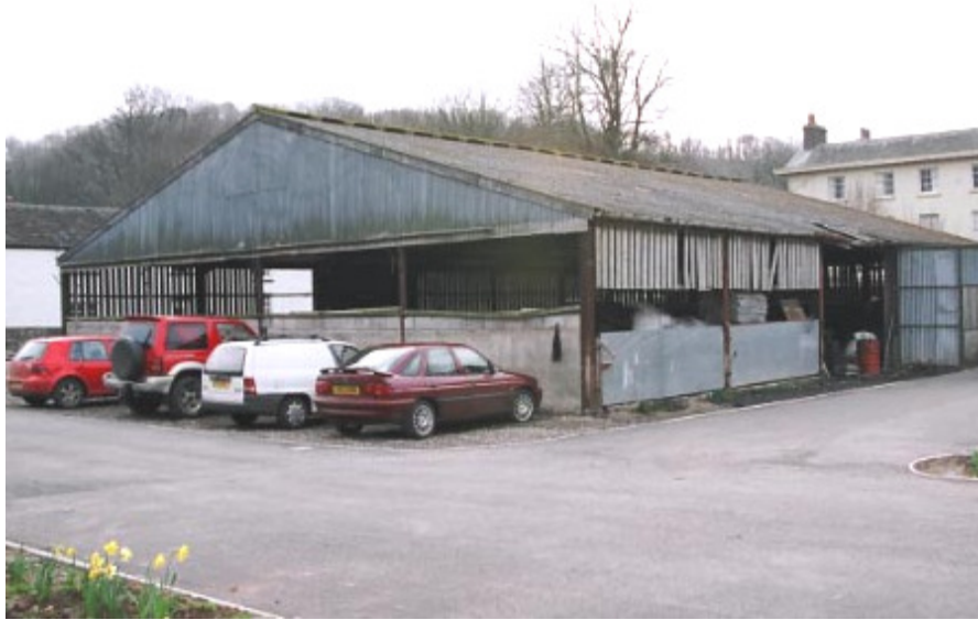
Fig. 1 Redundant Agricultural Building at Llancayo Court before conversion
