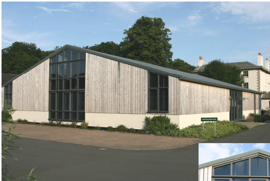
Fig. 2 Redundant Agricultural Building at Llancayo Court after conversion
