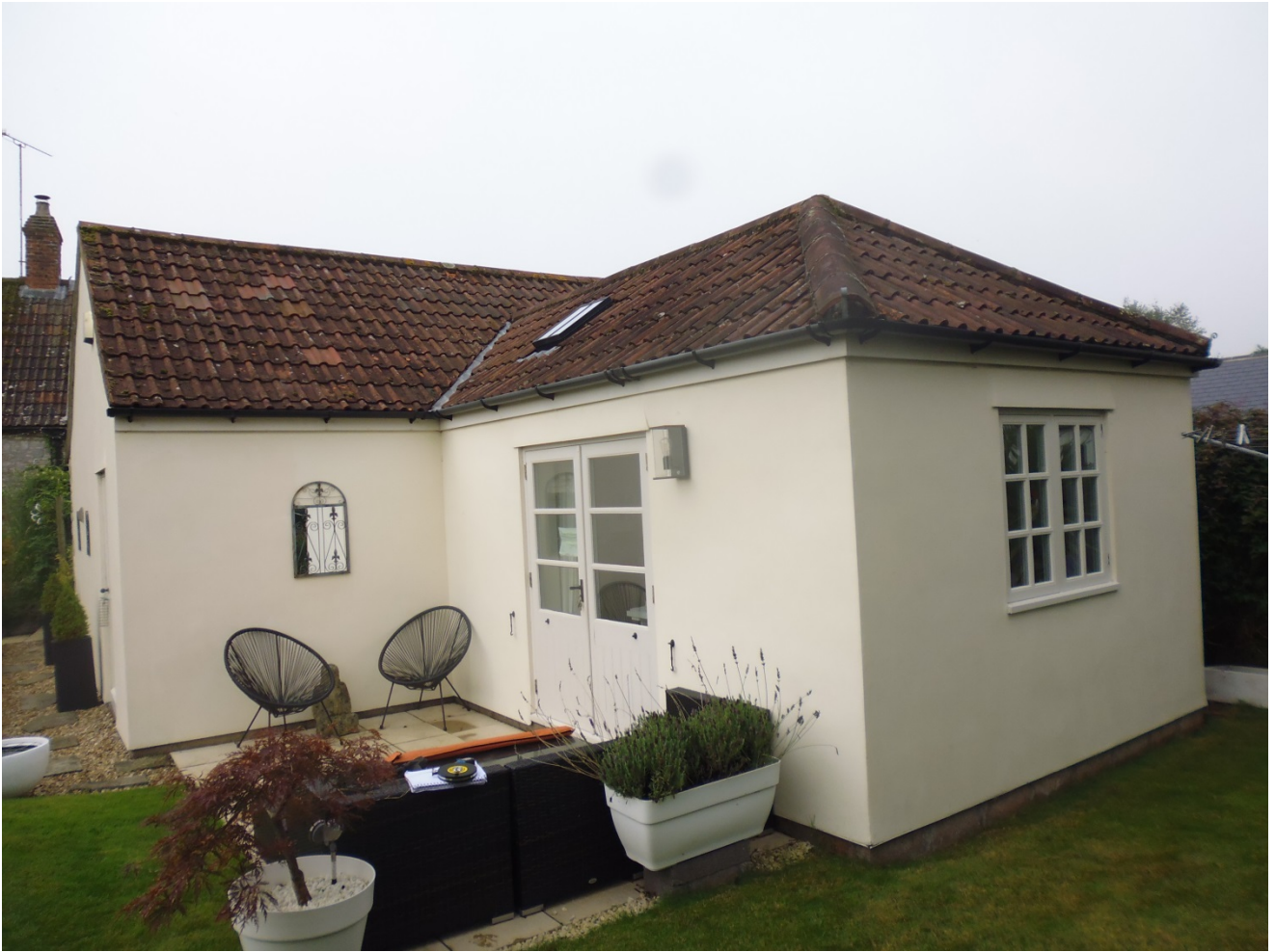
View of rear of existing garage building
