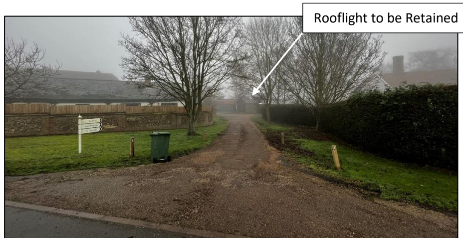
Rooflight viewed from the Highway
