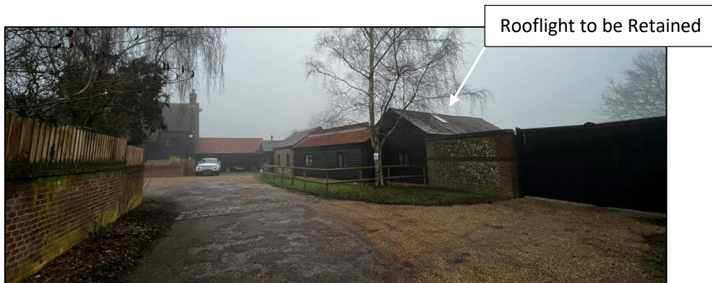
Rooflight viewed from the Shared Driveway
