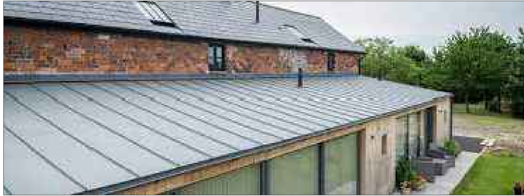
Image of Standing Seam Roof
