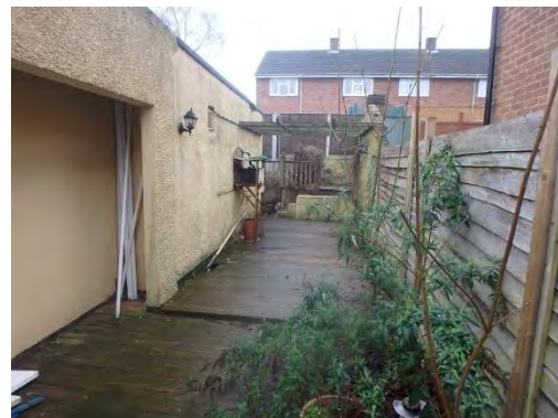
Photo 3 – view across rear of building
