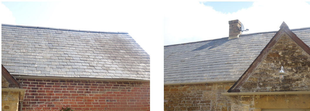
Figs. 3 & 4 Ridge and roof tiles
