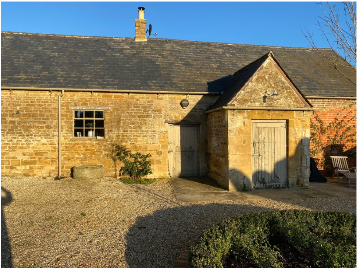
West elevation middle part
