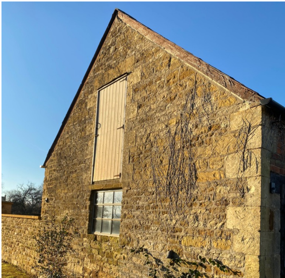
South gable detail
