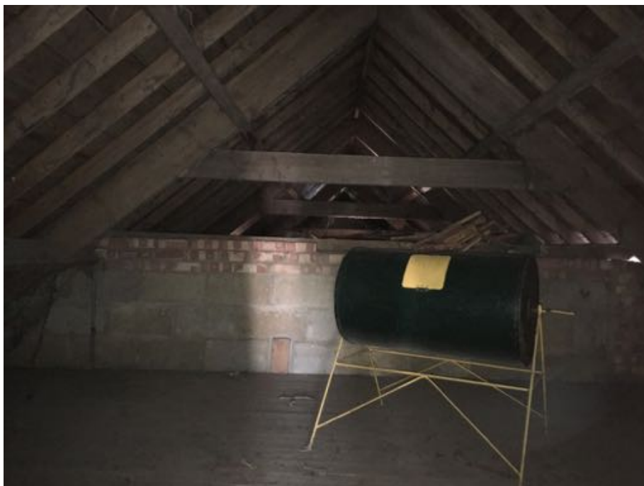
Above photo shows 'original' trusses in main section of stables.
