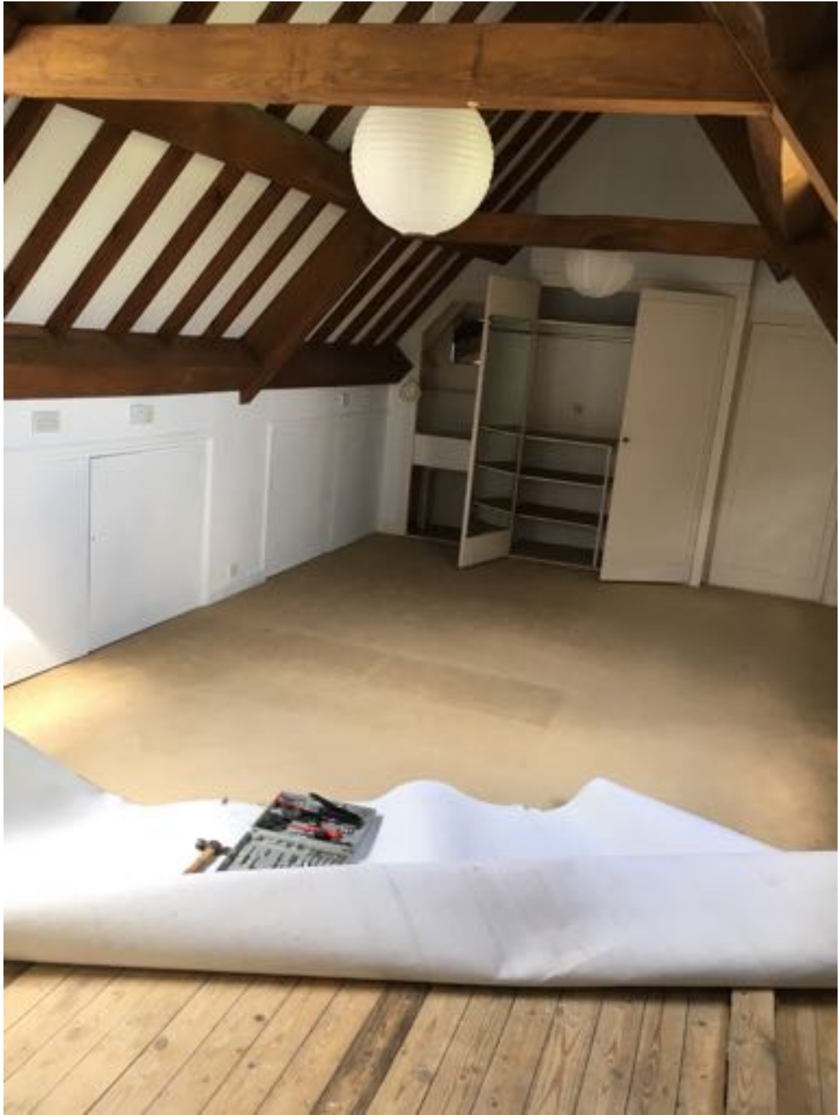
3.2 Note: photos above show modern rafters and trusses, and modern pine floorboards and modern joists.
