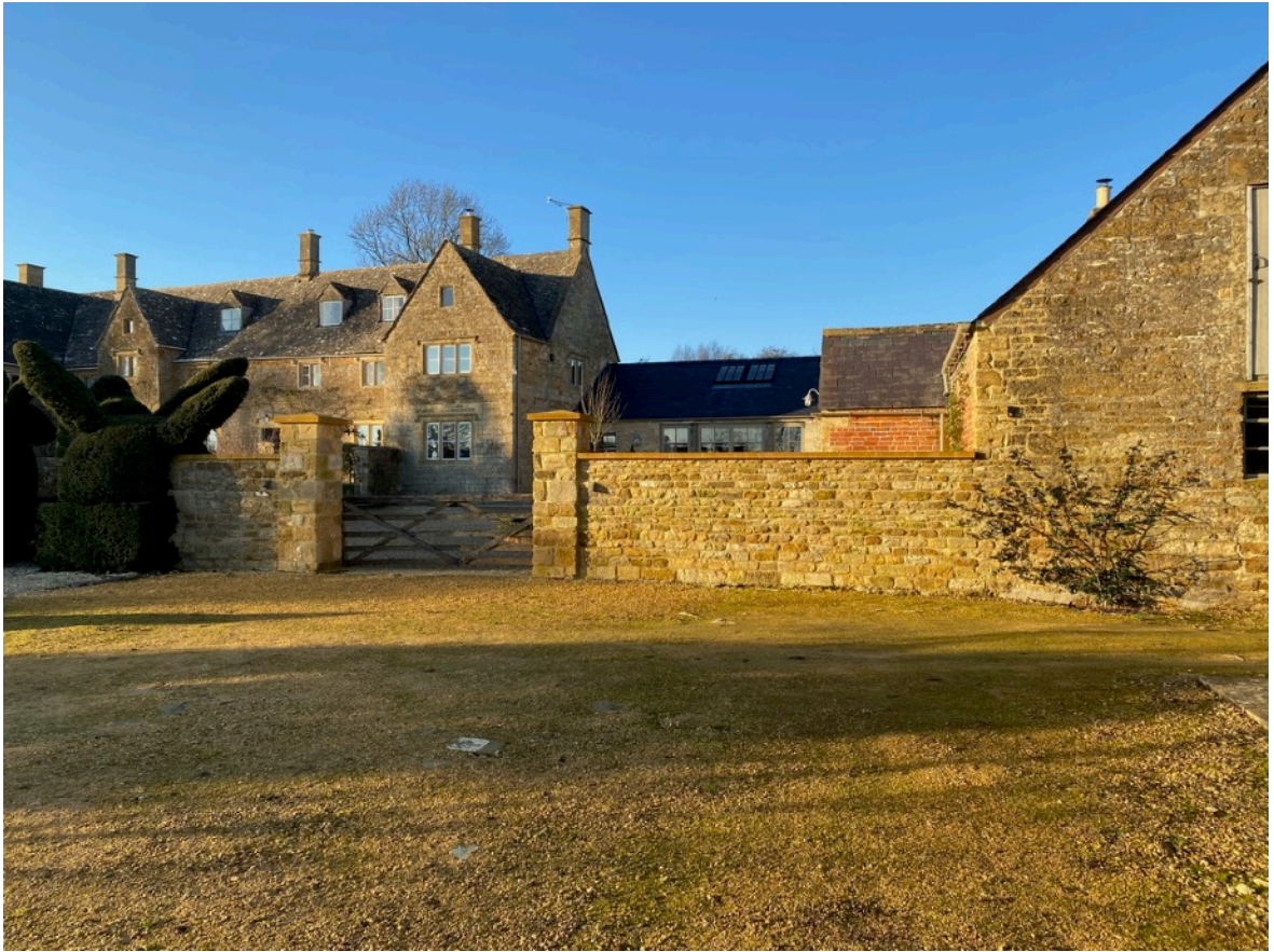
Rear garden wall left of South elevation
