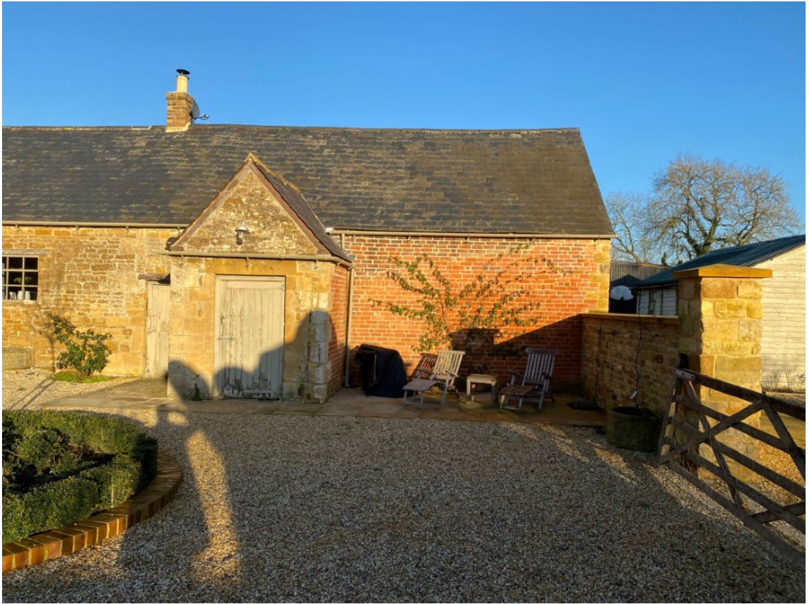
West elevation end
