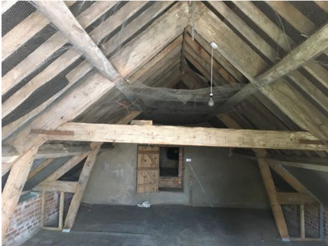
Above photo: truss from 'amended' south section of stables. Note clean bricks above eaves, and use of dropped chords to support the floor.
