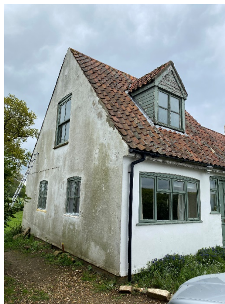
North side with existing two storey structure
