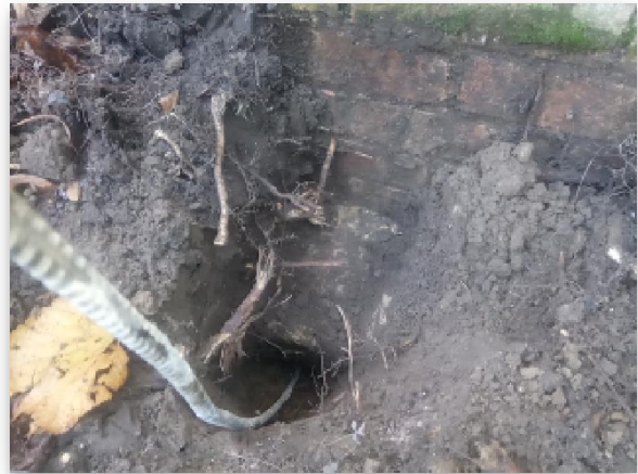
Fig 1.2: Trial Hole 1 Footing
