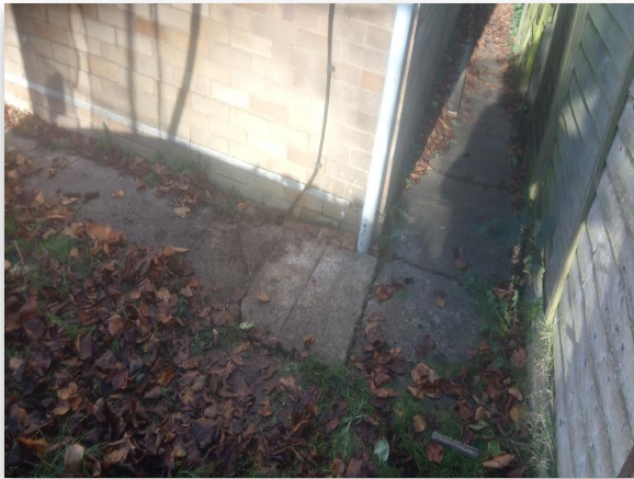
Fig 1.1: Trial Hole 1 Location
