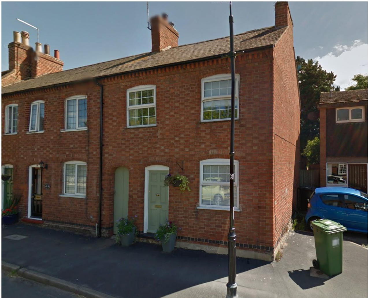
Photograph of the front elevation of the property
