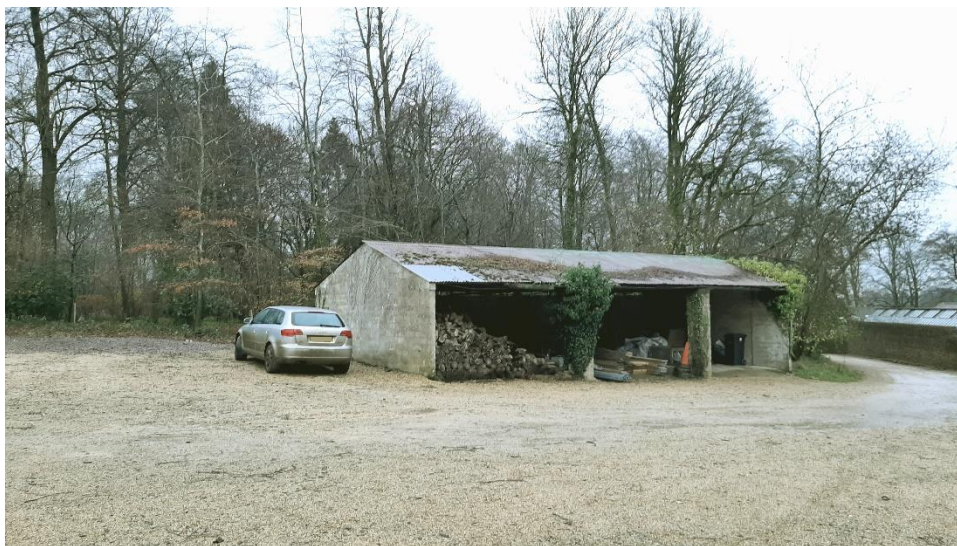
Site photo of Outbuilding B
