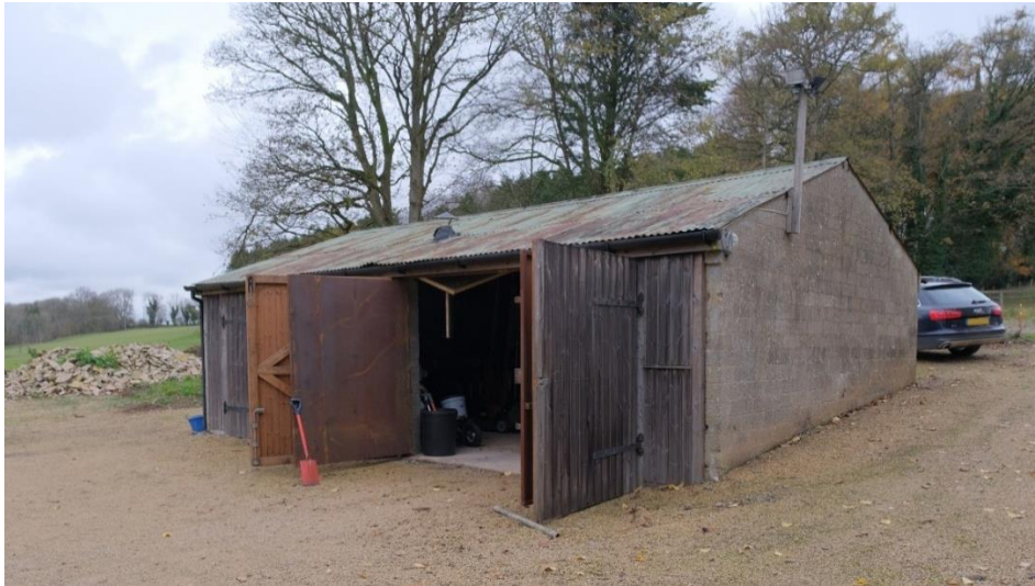
Site photo of Outbuilding C
