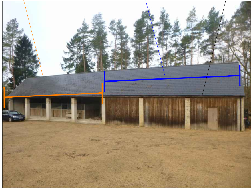
Photograph 1: Showing the eastern elevation for the barn.
