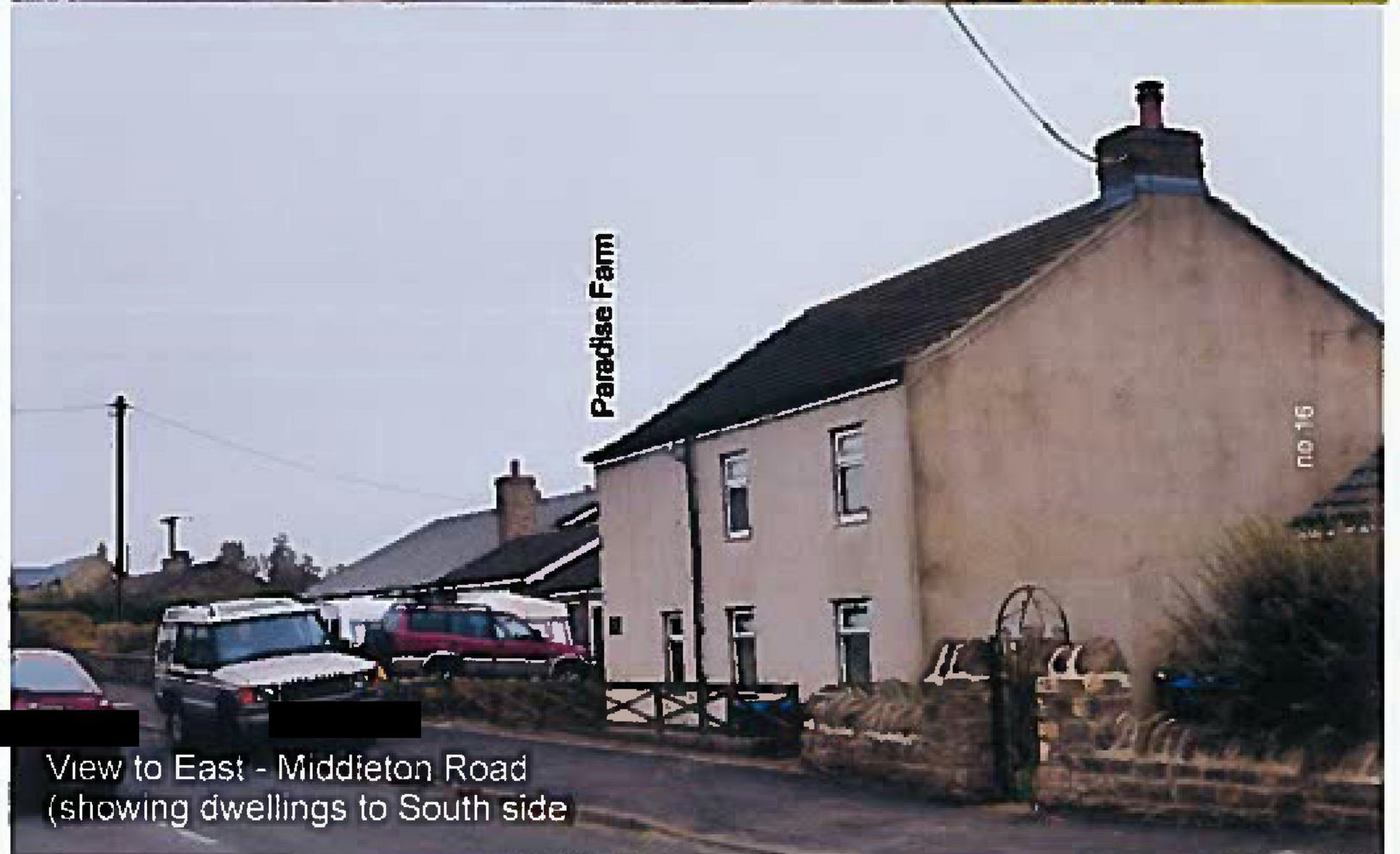
View to East - Middleton Road (showing dwellings to South side)
