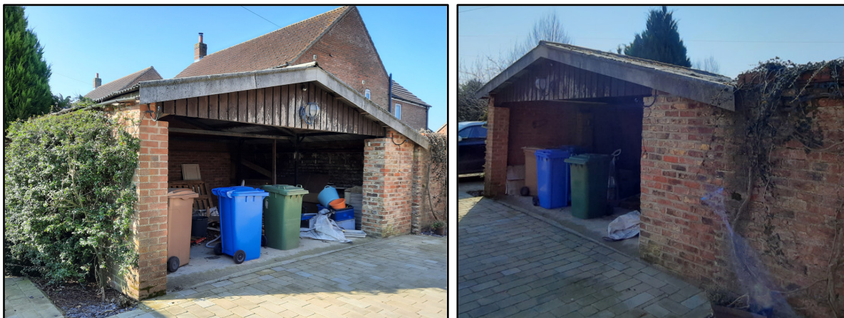
Plate 2 – Southern elevation wall showing the roof covering, and brick gutter supports.
