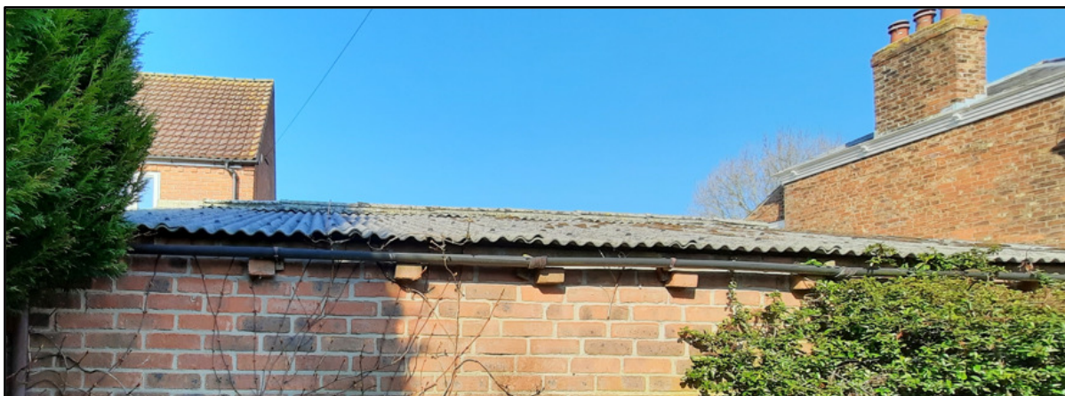
Plate 2 – Southern elevation wall showing the roof covering, and brick gutter supports.
