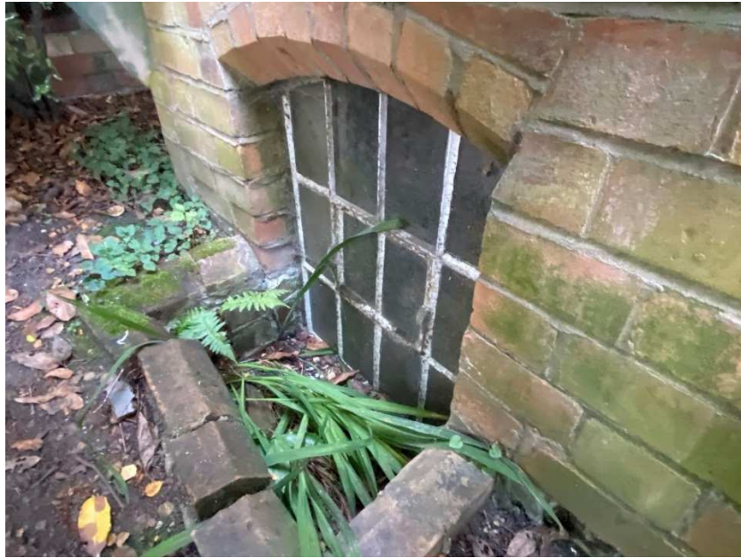
Existing basement window to front elevation
