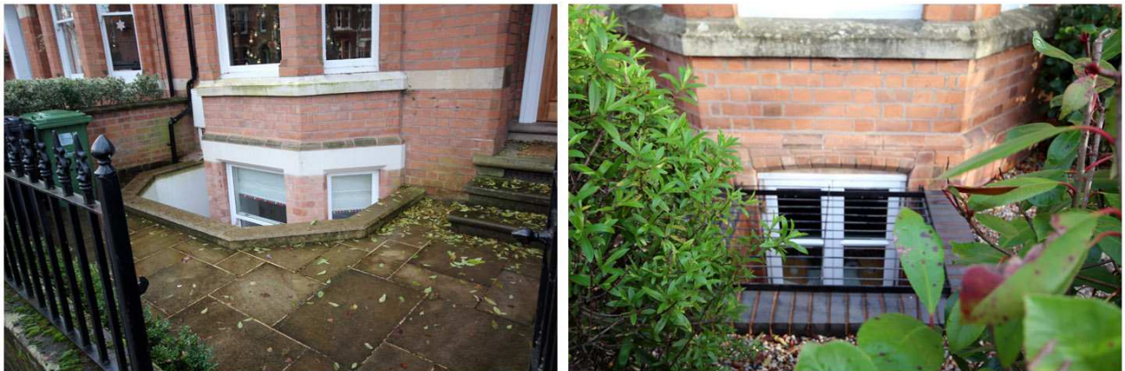
Example of escape lightwells along Gaveston Road
