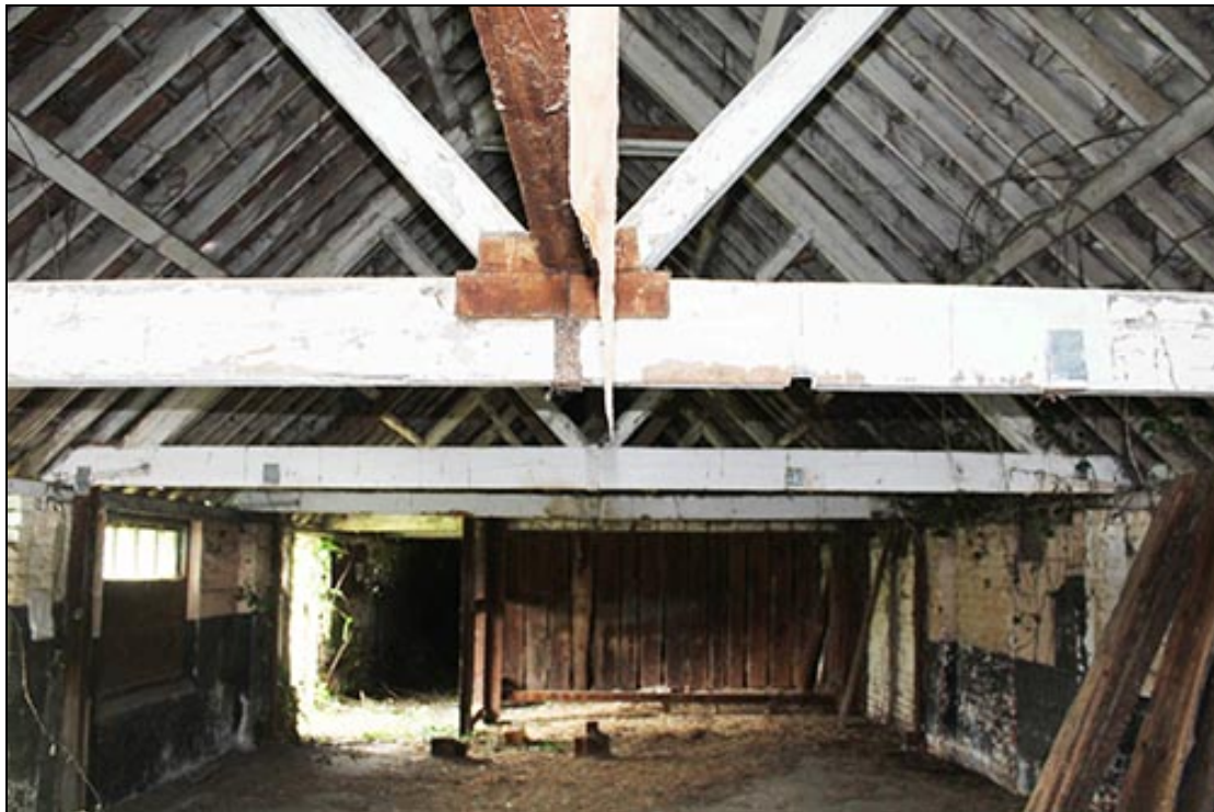
Figure 32 The central and western blocks of the Stables, looking east
