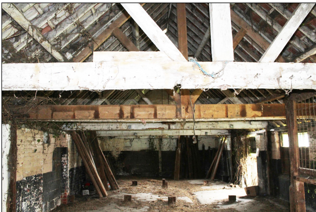
Figure 33 The central (western part) and western blocks of the Stables, looking west. The division between the two is marked by the new truss (not painted white) that was inserted in the late 20 th century.
