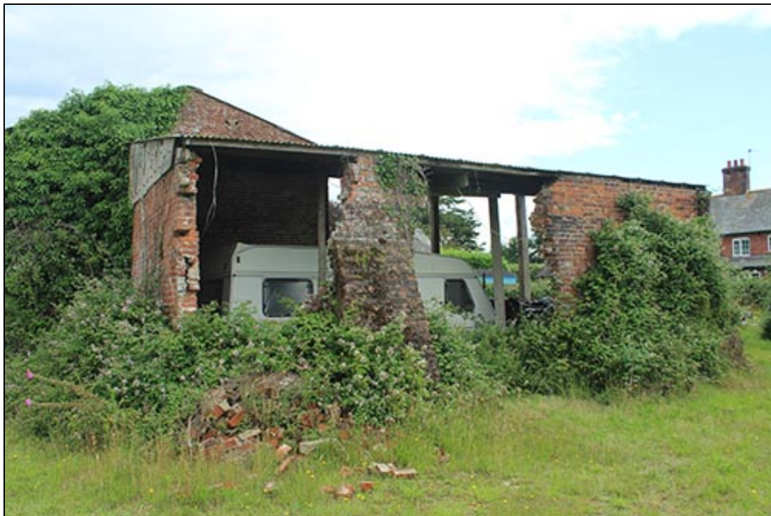
Figure 23 The Lean-to looking north-east
