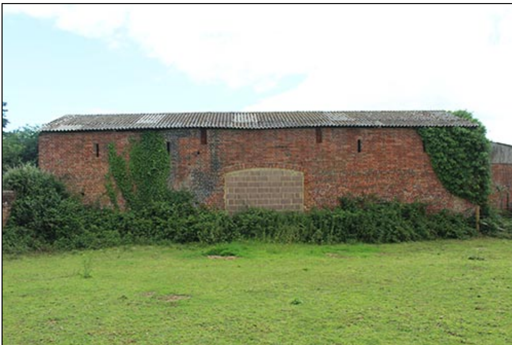
Figure 18 The west elevation of the Brick Barn
