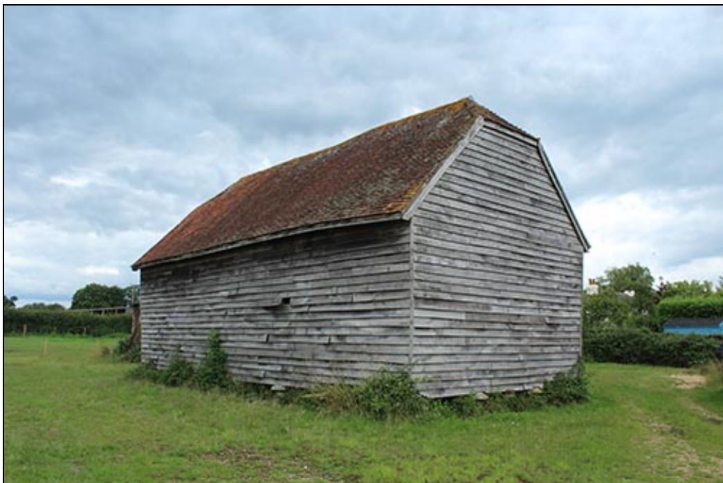
Figure 12 The Threshing Barn looking north-west
