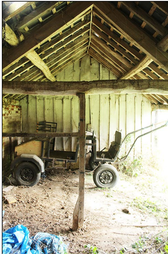
Figure 27 The interior of the Shelter Shed, looking east at the later partition inserted after the addition of the Small Store
