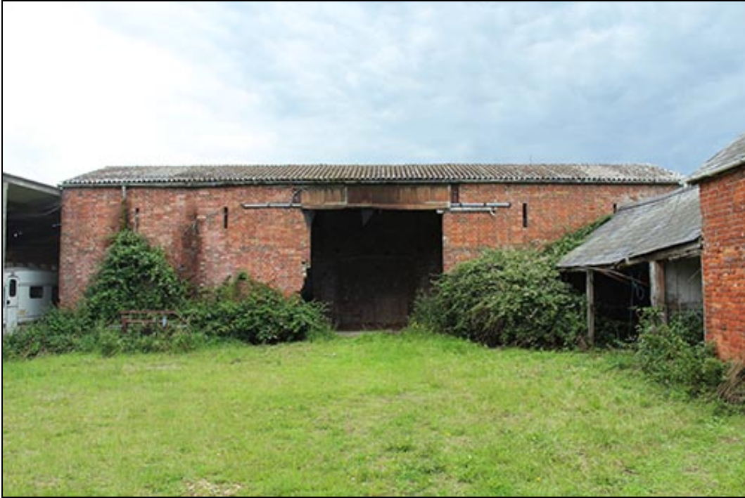
Figure 17 The east elevation of the Brick Barn
