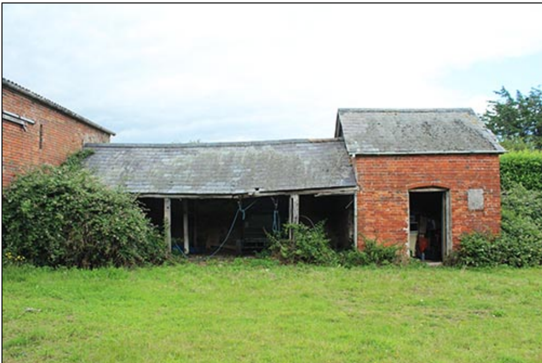
Figure 25 The Shelter Shed and adjoining Small Store, looking north
