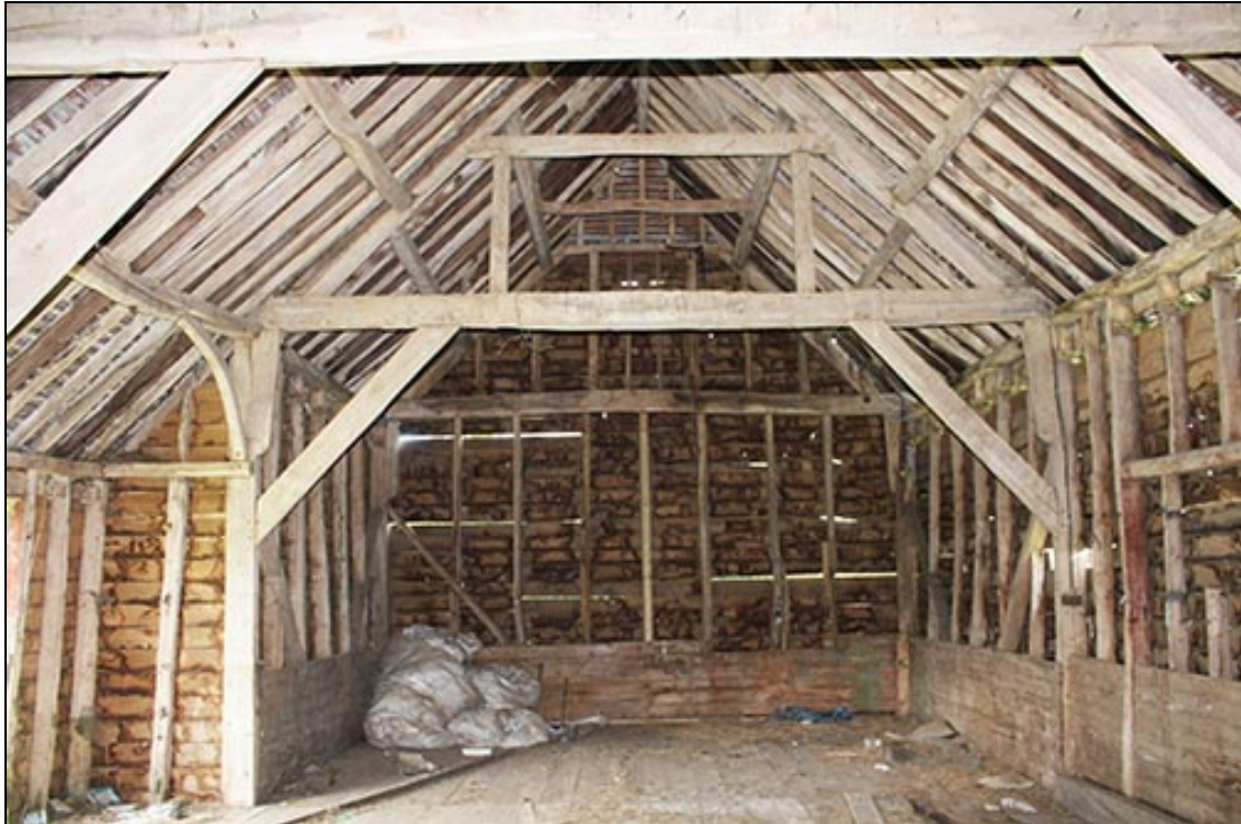
Figure 16 Interior of the Threshing Barn looking east showing the frame construction and the softwood boarding on the lower walls that replaced the earlier beech boards of the eastern bay in the late 19 th or early 20 th century. One of the additional collars between the purlins can be seen in the bay roof above, as well as the additional rafters. To the left can be seen one of the arch braces and the timber affixed to the soffit of the northern porch
