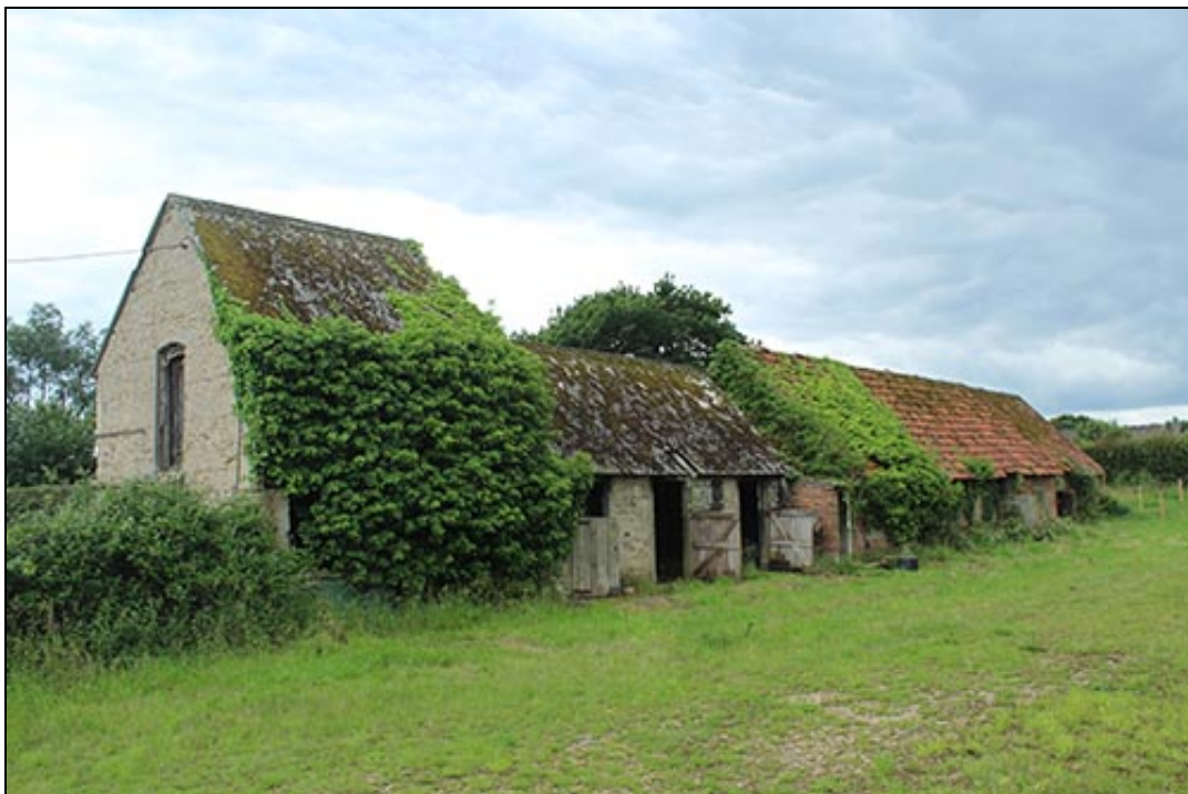
Figure 30 The Stables and Large Store looking south-west
