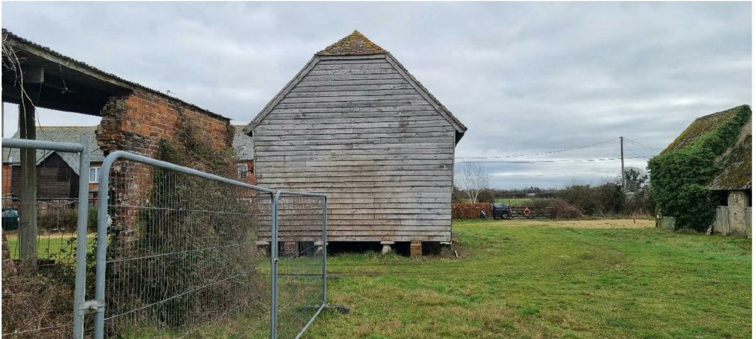
Barn B – Western elevation
