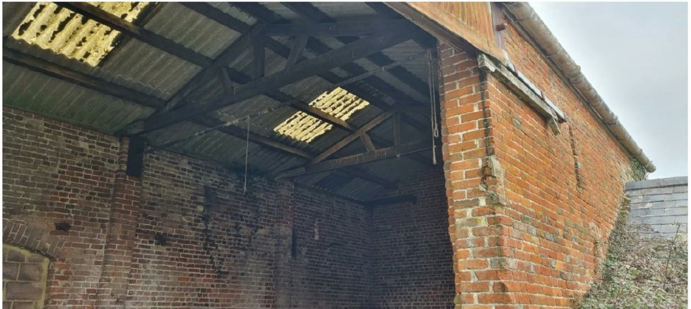
Barn A – Eastern elevation showing the connection to Barn C
