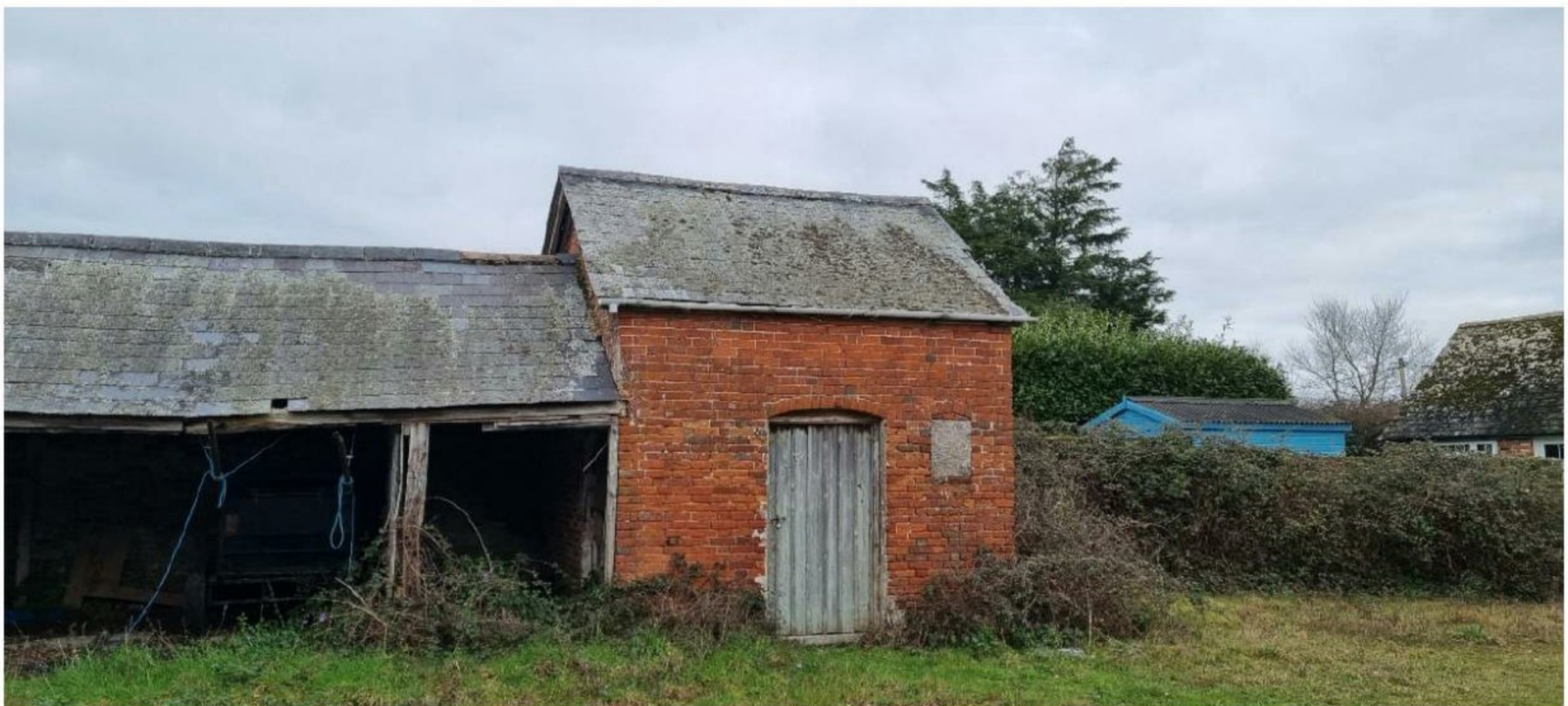
Barn C – Southern Elevation
