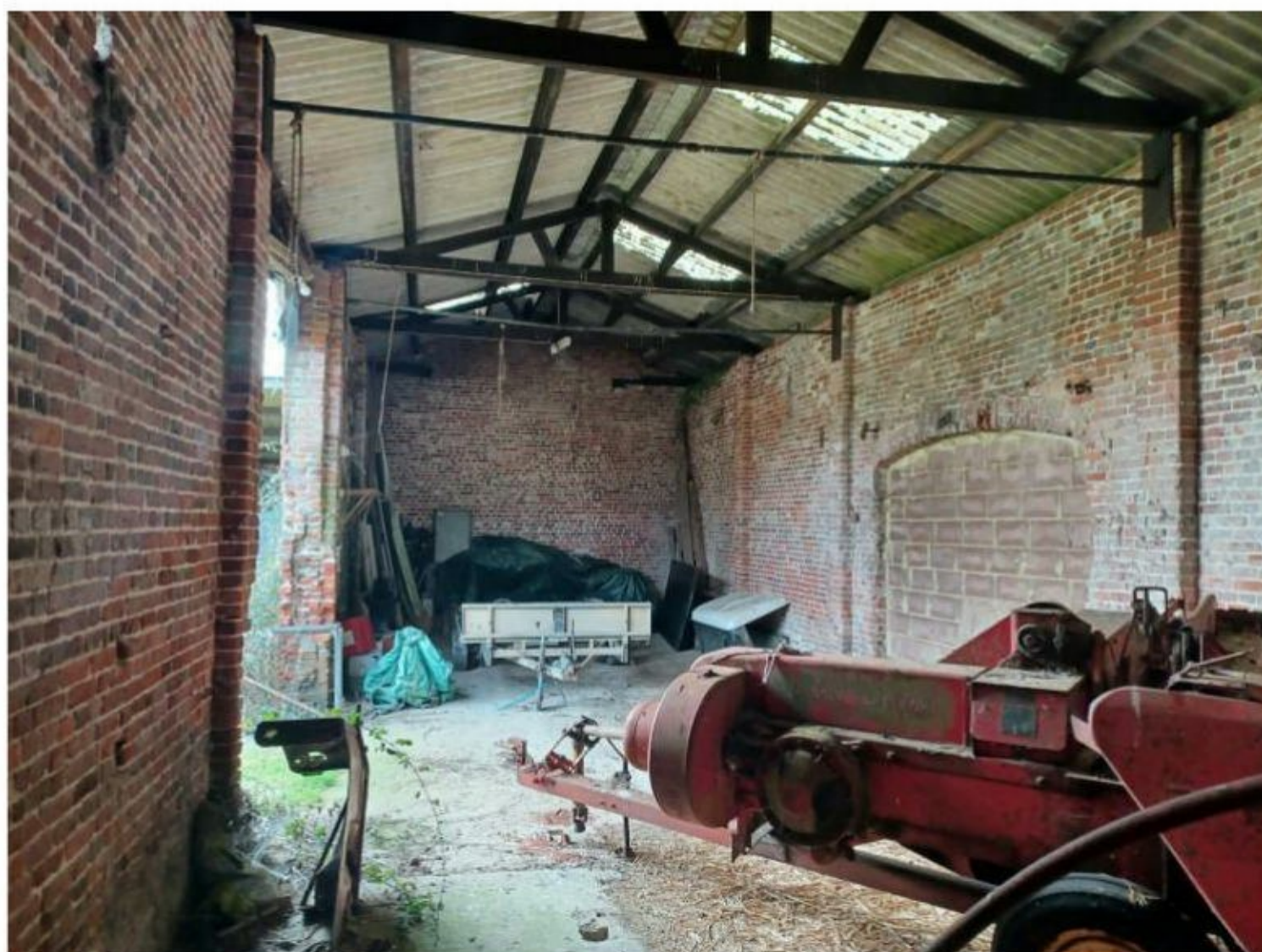
Figure 3 - Main Building (Internal)
