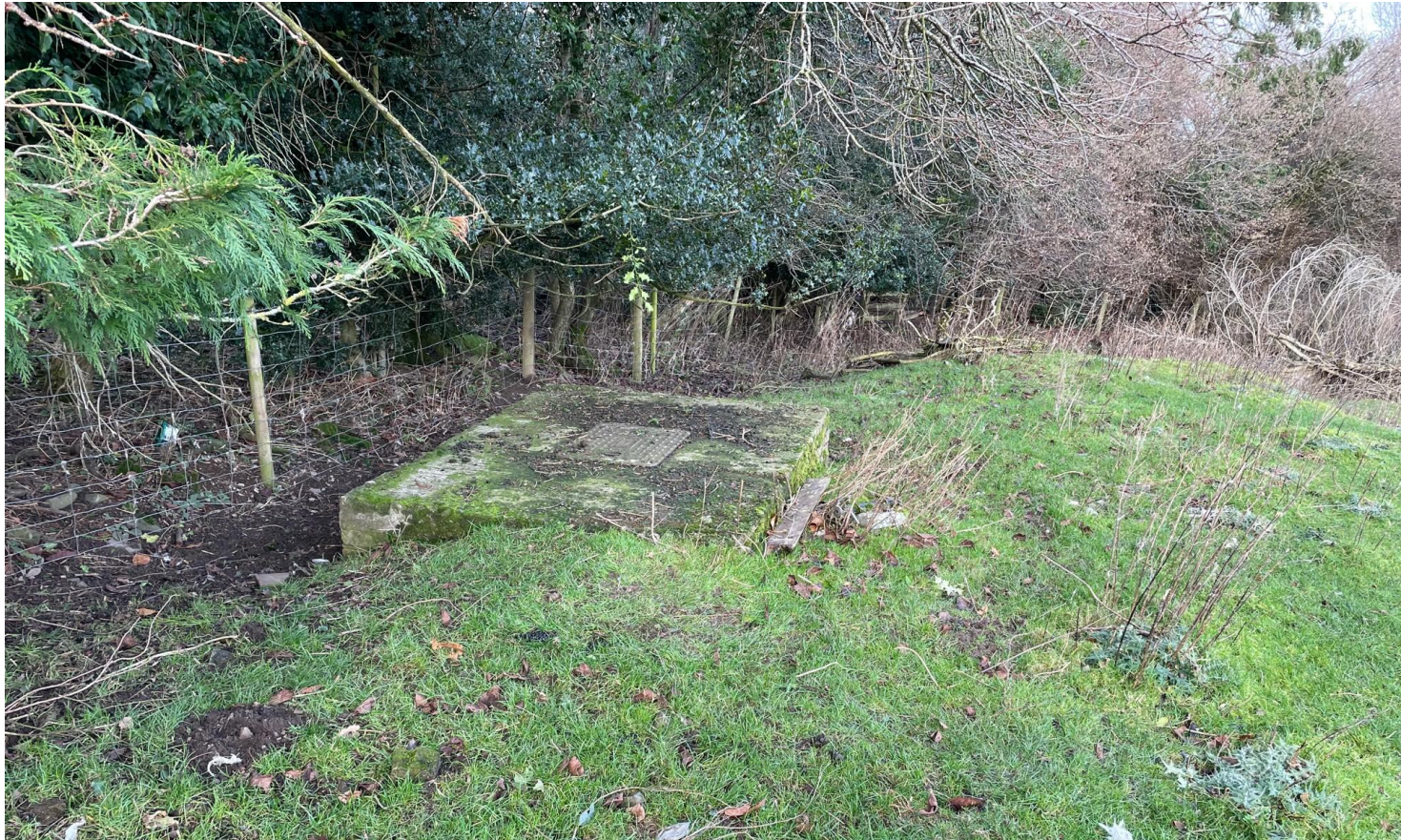
Existing Septic Tank
