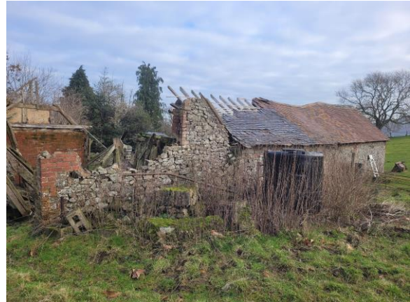
P2: Building A: W + S elevations, viewed from the SW
