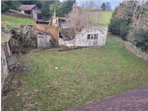
P7: Courtyard area to the N, looking NW
