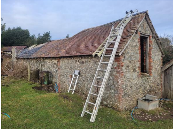
P1: Building A: S + E elevations, viewed from the SE
