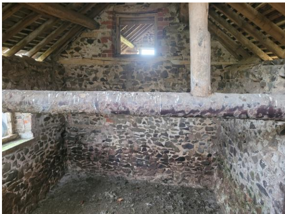
P3: Building A: Interior, W-end; looking E
