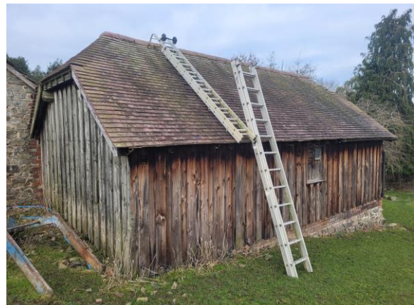
P4: Building B: S + E elevations, viewed from the SE
