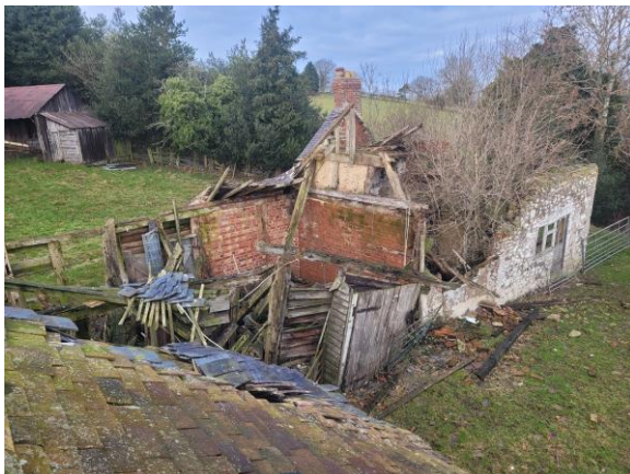
P5: Building C: E elevation, viewed from the SE
