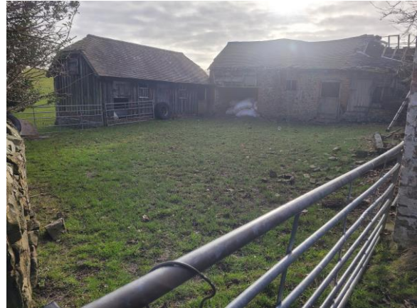
P8: Courtyard area to the N, looking SE
