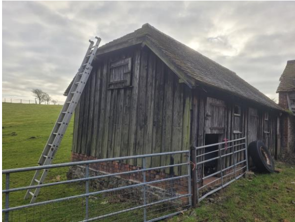
P5: Building B: N + W elevations, viewed from the NW
