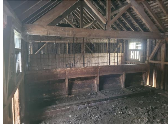
P6: Building B: Interior, S-end; looking N
