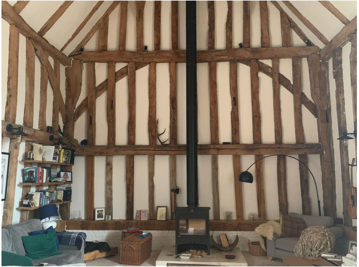
Internal view of barn showing North elevation
