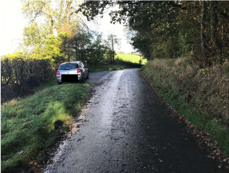
Location 1: localised widening at access, tarmac construction.
