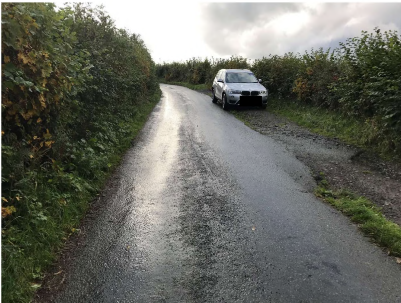
Location 8: informal stone passing bay at farm access track.
