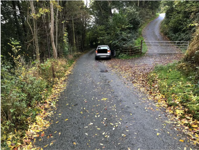
Location 9: localised widening at access, tarmac construction.
