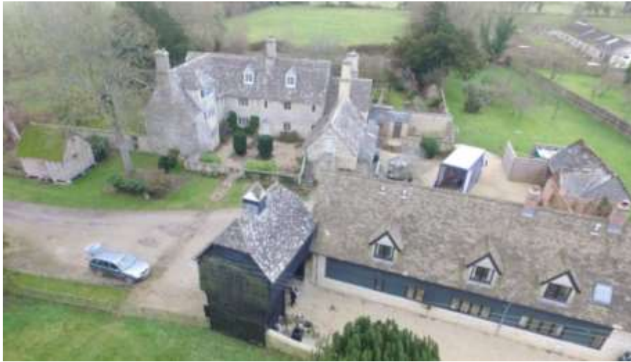
Aerial view of the group of buildings with Extra Cover to the front of the picture
