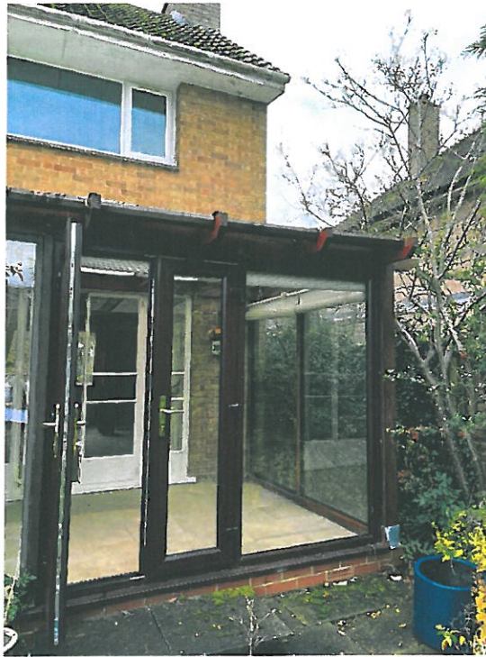
Fig. 7 Photo showing existing conservatory structure
