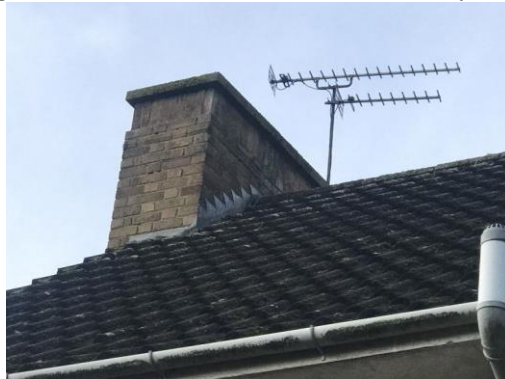
Image 3: B1 viewed from east side. Close up on roof
