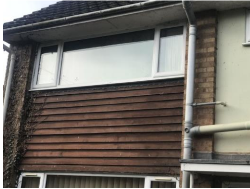
Image 4: B1 viewed from east side. Close up on cladding
