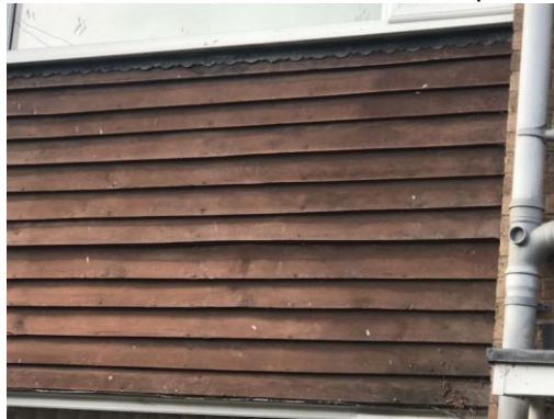
Image 5: B1 viewed from east side. Close up on cladding
