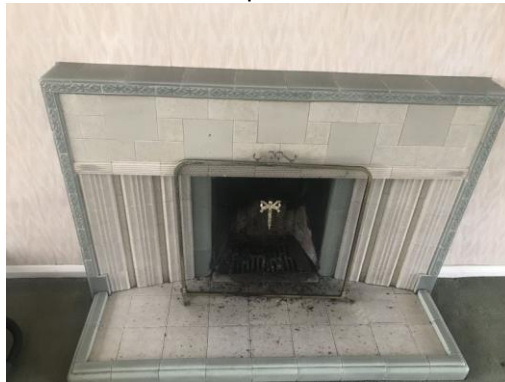
Image 26: B1 interior. Fireplace connected to chimney
