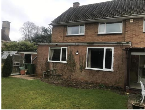
Image 13: B1 viewed from west side
