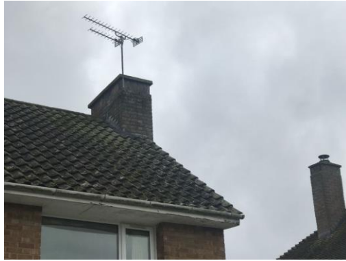
Image 16: B1 viewed from west side. Close-up on roof
