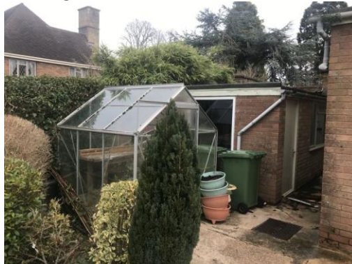
Image 27: B2 viewed from west side
