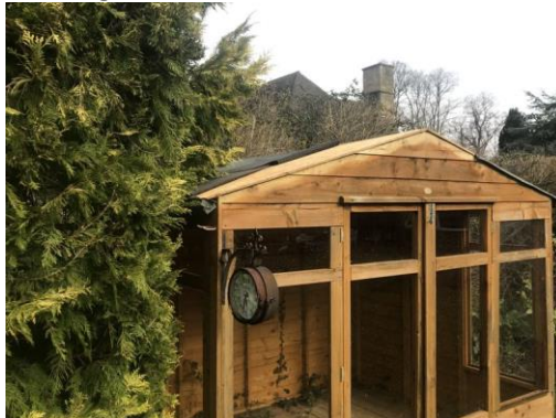
Image 36: B3 viewed from west side
