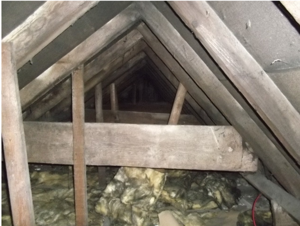
Plate 10. The roof void over the southern part of the public house
