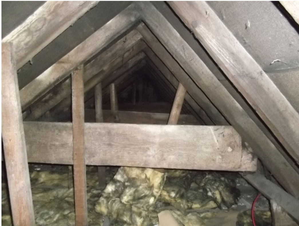
Plate 6. The roof void over the southern part of the public house
