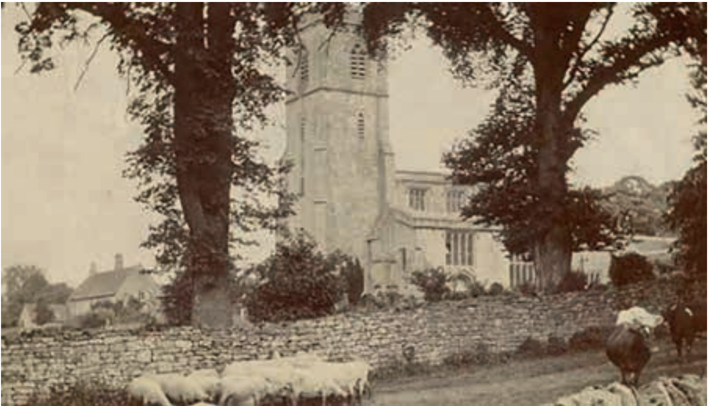
Collectively, Taynton's stone buildings form a recognizable and distinctive vernacular style of architecture that communicates its affinity with the traditions of the local context... They reflect a broader homogeneity in the regional character of the Windrush Valley defining the 'stony landscape' observed across villages such as Asthall Swinbrook, Widford and Burford (almost all which had their own quarry) by 20th century travellers such as J. Massingham.
