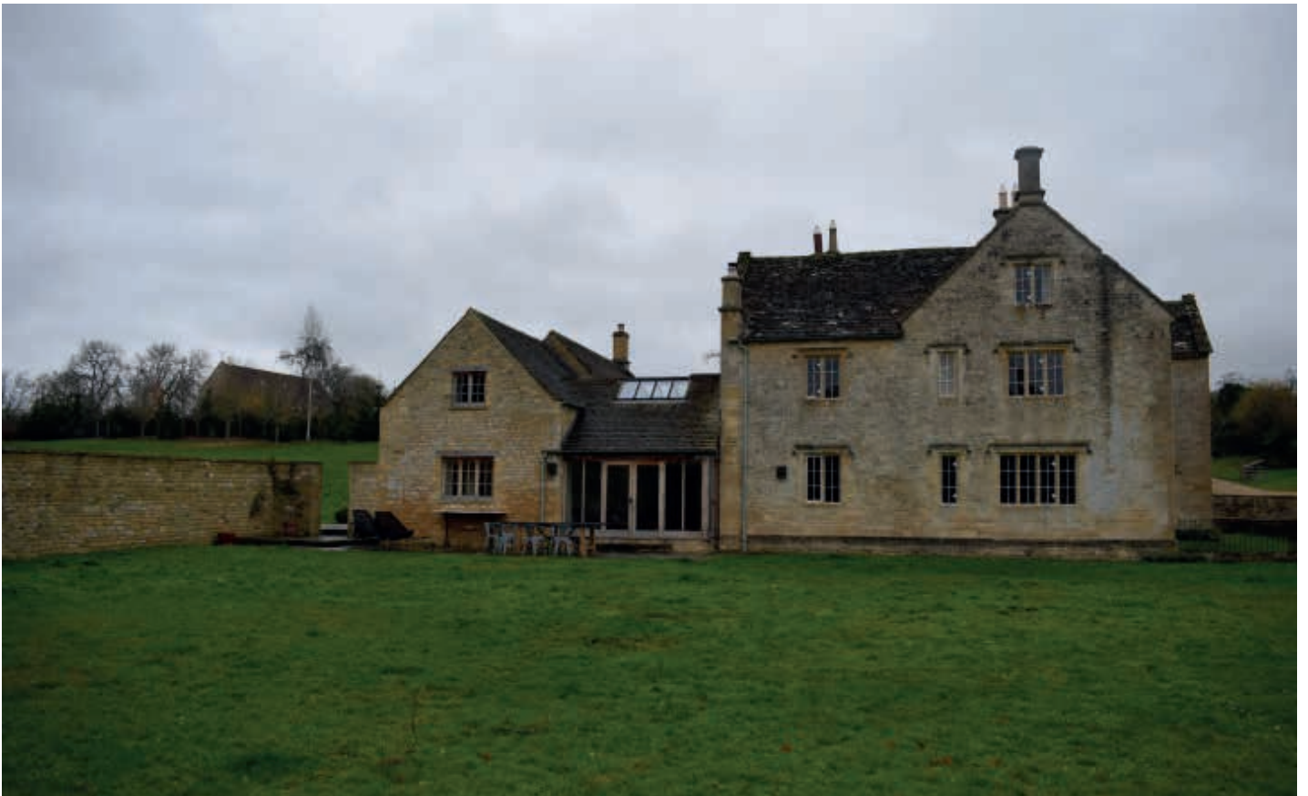
East side elevation with modern link noted in the planning images above
