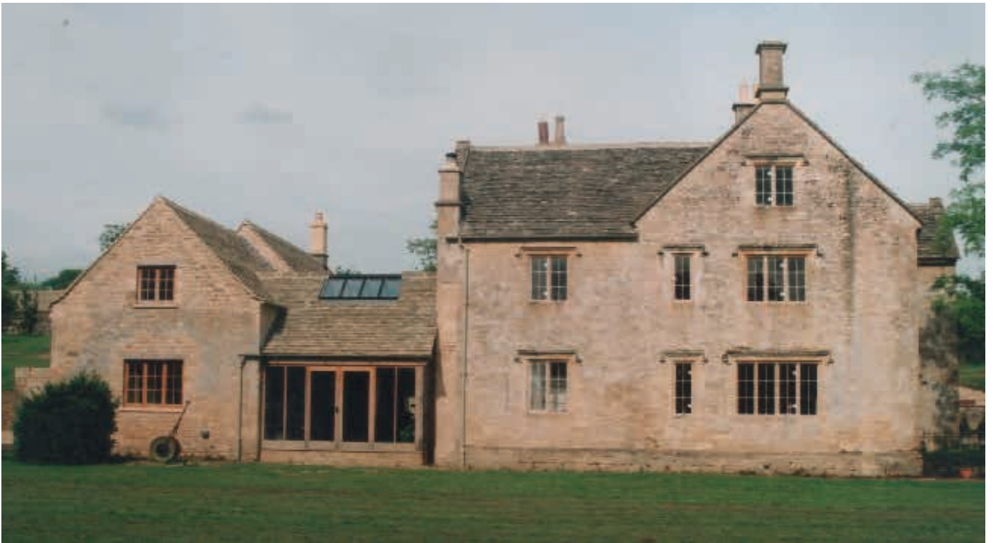
Image (undated) from Calder Architects website showing side elevation following works
