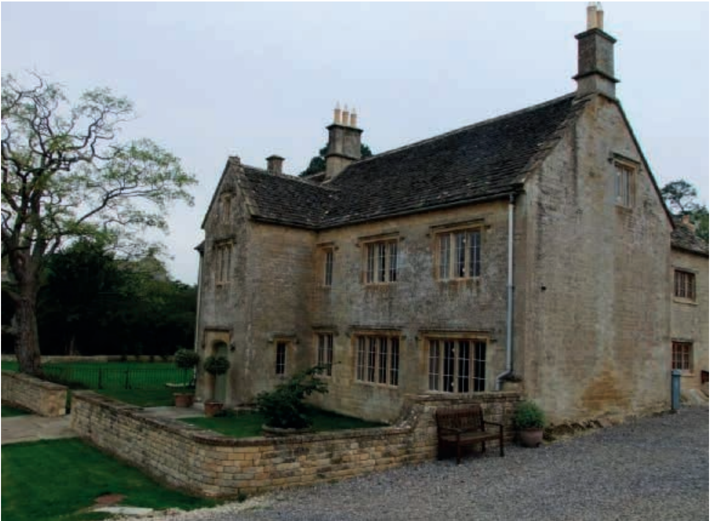
Front (south) and side (west) elevation of the house
