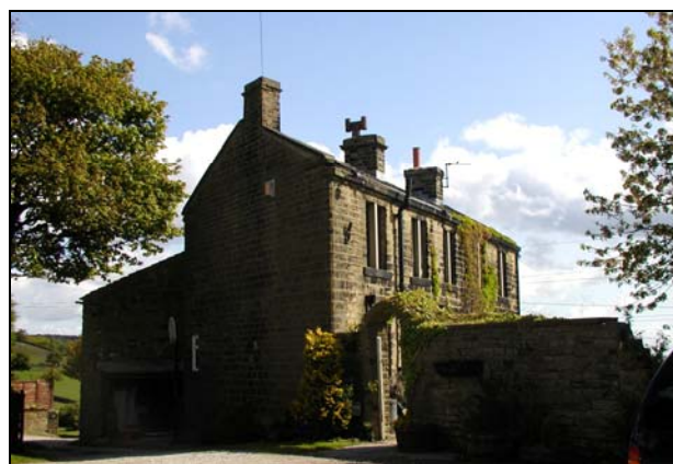
18 Ryecroft (Edge House) has an interesting chamfered elevation to the lane.
