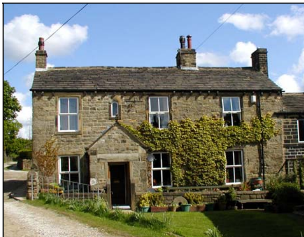
14 Ryecroft is an early to mid-19 th century house constructed of local stone with a stone slate roof.
