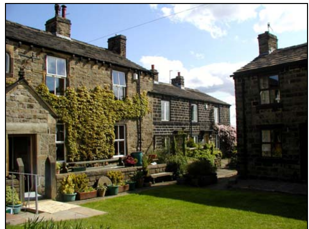
12 and 14 Ryecroft close off the northern side of the 'green'.
