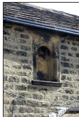
A stone arched recess above the main entrance.
