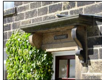
The stone corniced door case of 3 Ryecroft is a good example of where stone has been used for the decoration of buildings.
