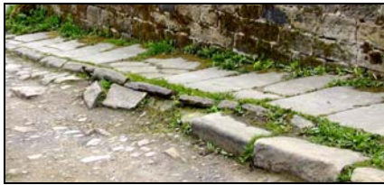
A small area of stone paved path alongside 5 Ryecroft.
