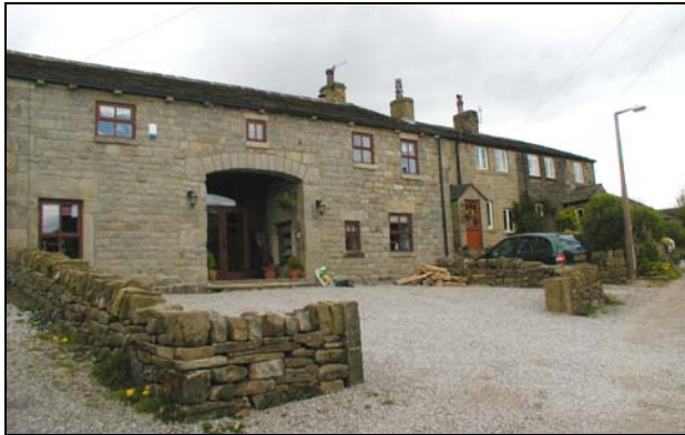
The barn (Grade II listed) has been converted into a dwelling in recent years. To the north are two cottages, 23 & 25 Ryecroft.
