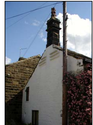
Projecting ledges on the west elevation indicate pigeons were once housed in the loft space.
