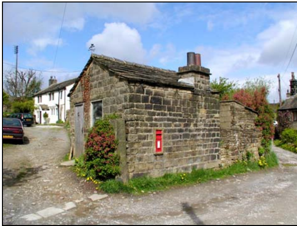
This interesting building appears to have had many uses in the past, such as a workshop, garage and possibly even a shop.
