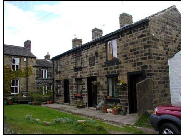
6-10 Ryecroft. Above the doorway to no. 8 are two stone carved heads to either side of date panels.
