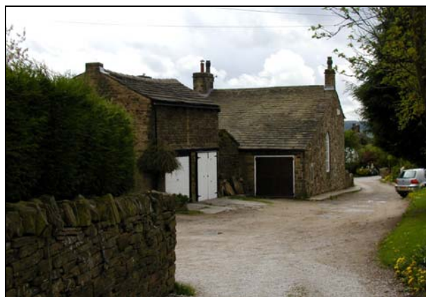
The outbuilding to the north of 14 Ryecroft has prominent white garage doors that overpower its simple character.
