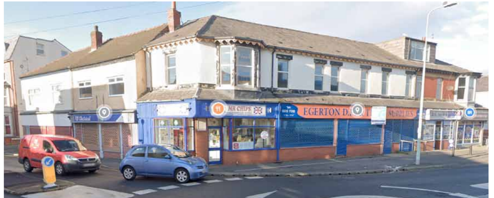
113-119 EGERTON ROAD - CORNER OF PLEASANT STREET AND EGERTON ROAD
