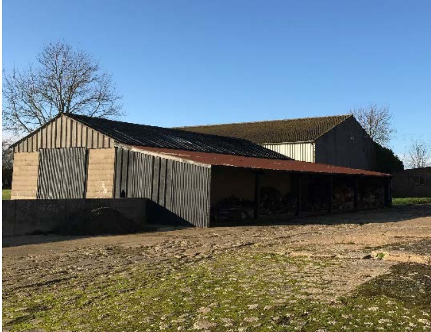
Front elevation of the barn as existing
