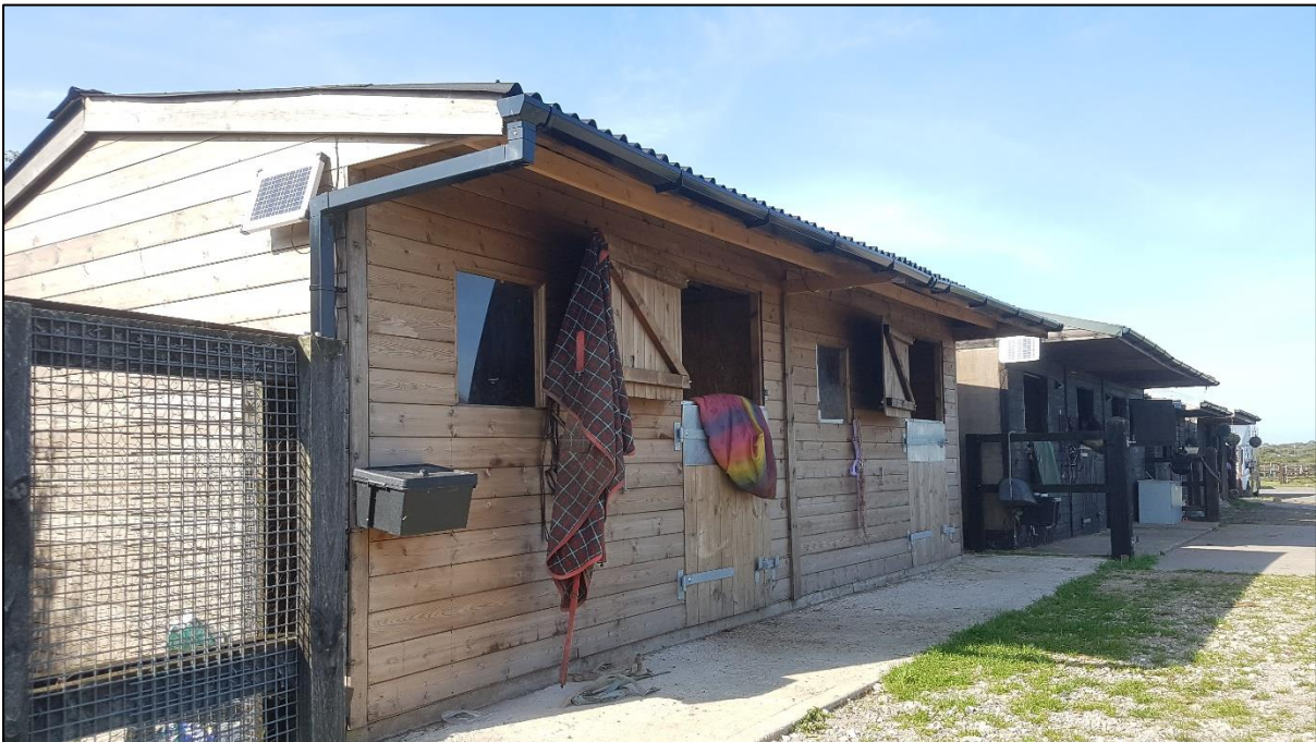
Plate 10: The Stables had single-skin corrugated sheet roofs.
