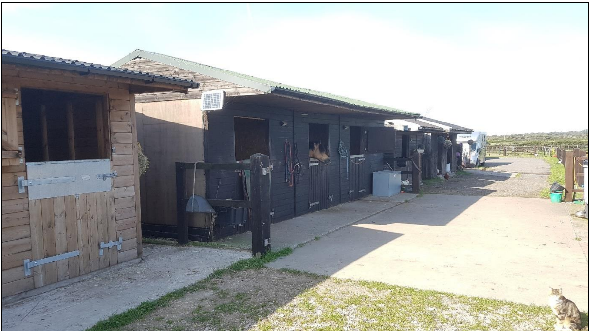
Plate 8: Hardstanding covered some parts of the ground adjacent to the stables/loose boxes.
