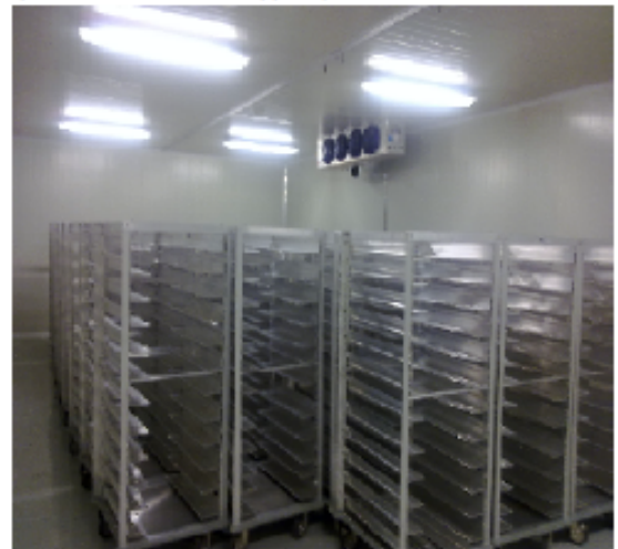
Chiller room, Evaporator installation with ceiling suspension system.
