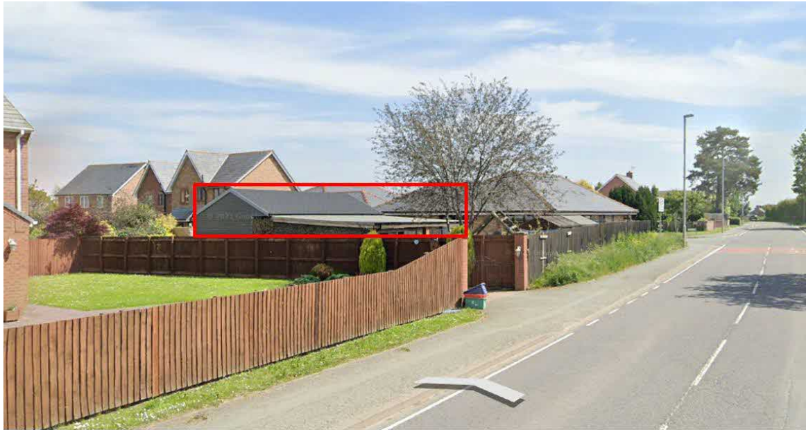
View of the site when directly adjacent, again showing the building with the context of the host dwelling and surrounding properties:
