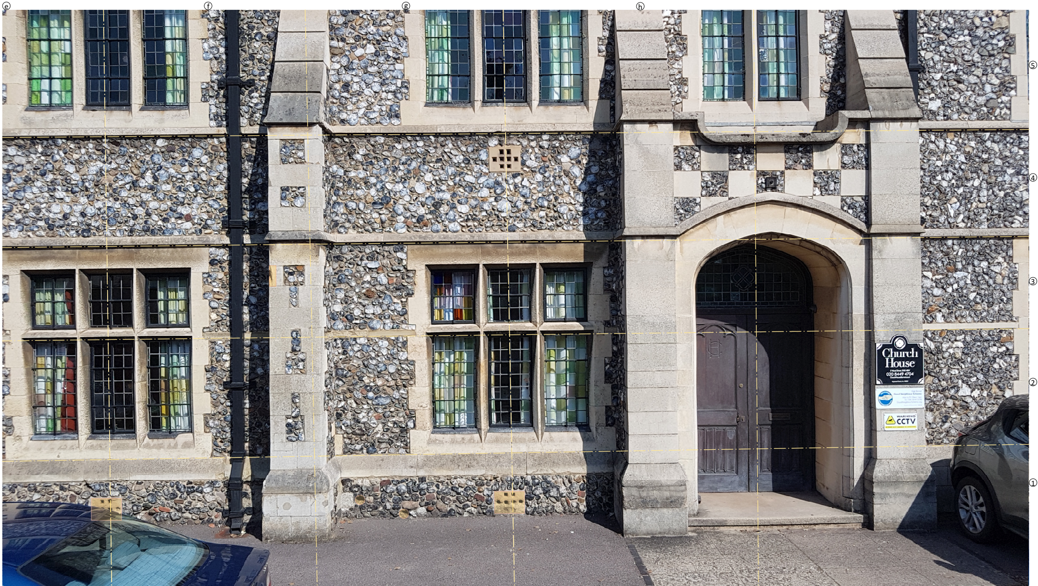
damaged face to buttress quoin (poorly bedded bath stone)
