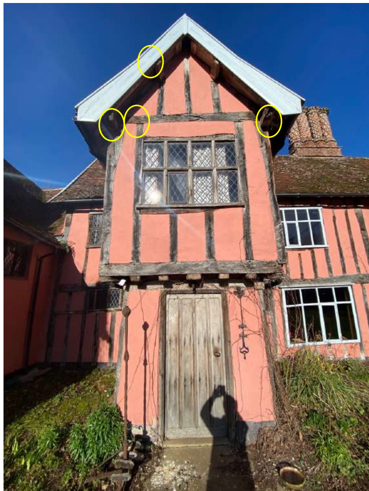
Photo 3 – Features above the porch where bats were observed emerging from.
