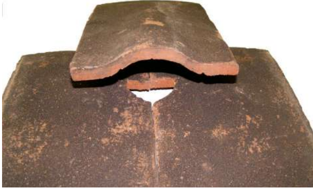
Photo 8 – an example of a bat access roof tile
