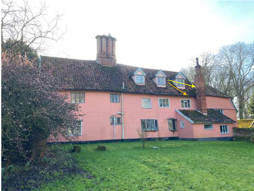
Photo 2 - Locations of emerging common and soprano pipistrelle bats from the northern elevation of Monks Hall at 21.47 on the 9 th of June 2021.
