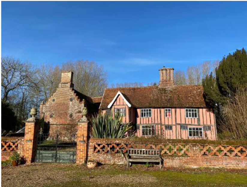
Photo 1 – Southern elevation of Monks Hall
